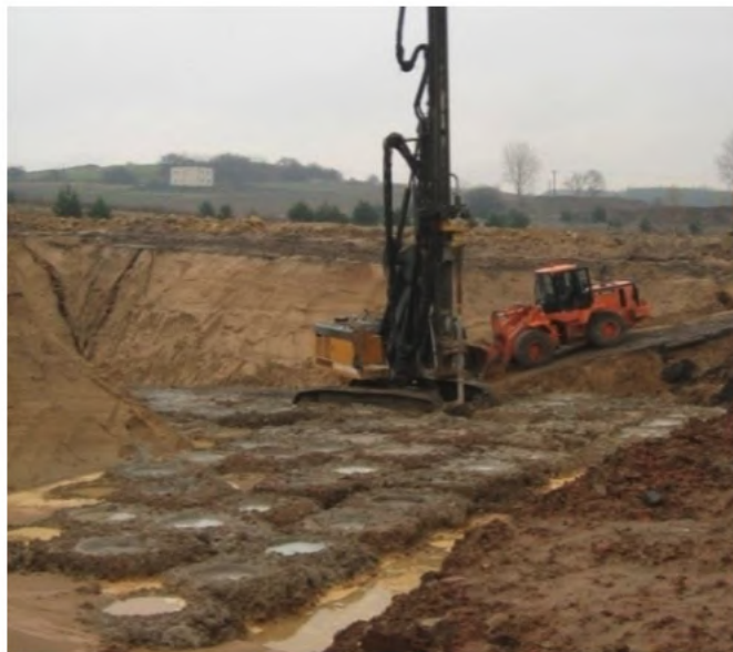
Figure 5-2: Methodology of soil mixing (Topolnicki, 2016)
