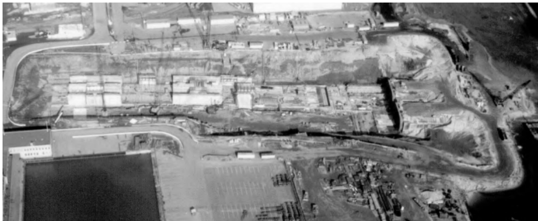
Figure 2-20: West cofferdam Fort McHenry tunnel. Tunnel elements with closure dike on right (Grantz, 2001)
