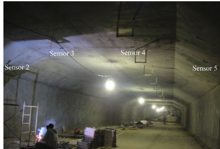
Figure 4-5: Field installation of FBG sensors (Wei et al., 2018)
