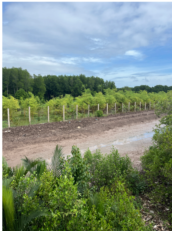
Figure 2.11: Earthen dike separating natural mangroves from mangrove integrated fishponds
