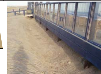
4.13 Hole creating effect by convection at the bottom of the facade
