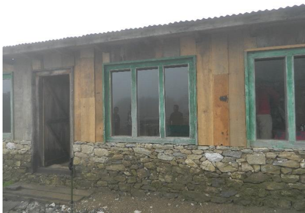
Figure 6.14. Timber framed house, with a mountain stone foundation (Shock Safe Nepal group 1).
