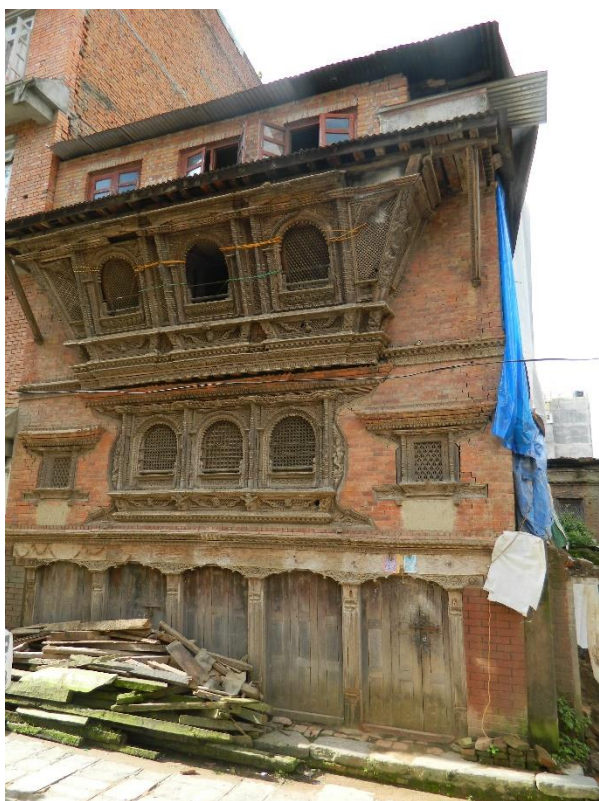
Figure 6.4. Low strength brick masonry house (Shock Safe Nepal group 1).
