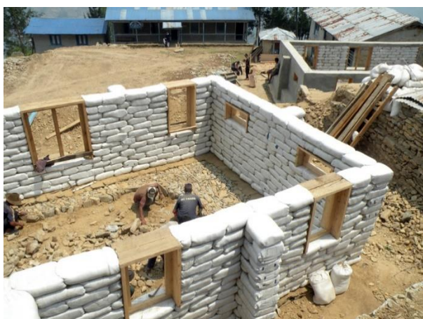
Figure 6.28. Construction of a house built with earthbags (Goodearthnepal, 2014).
