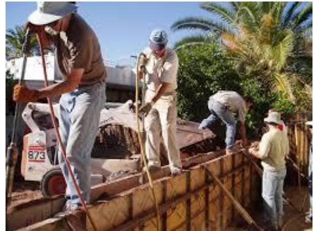
Figure 6.18. Construction work of a rammed earth wall (Wentworth designs, 2009).
