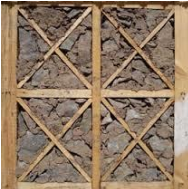
Figure 6.17.: Timber frame filled with mountain stone (worldhousing, nd).
