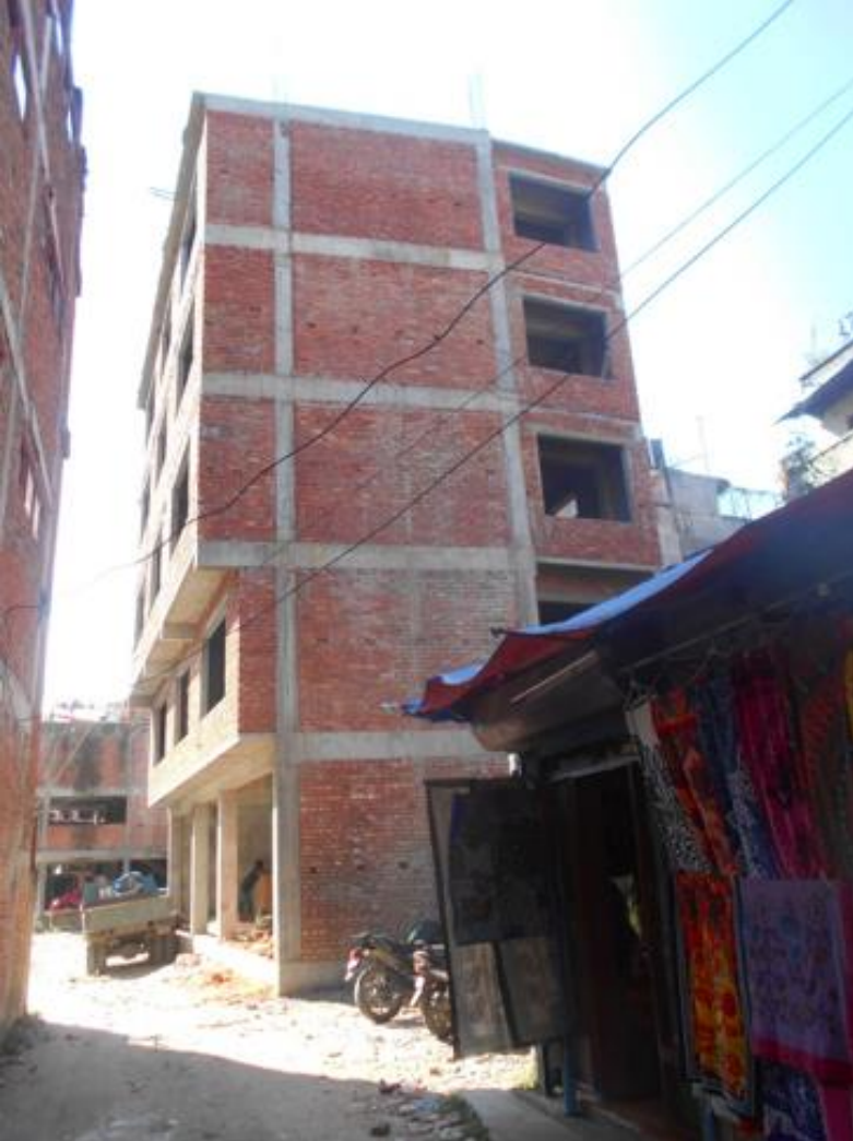
Figure 4.3. RCC building with discontinues load path (Shock Safe Nepal group 1).
