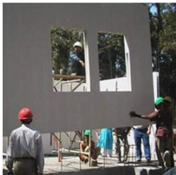
Figure 6.35. Construction of a house with Rapidwall panels. (greencross, nd).
