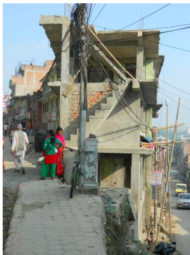
Figure 4.7. Uncontrolled RCC-frame buildings with unequal column lenath
