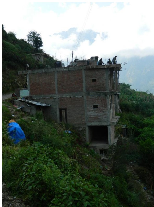
Figure 6.12. Reinforced cement concrete frame with brick infill house build on a slope (Shock Safe Nepal group 1).
