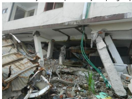
Figure 7.27: Soft story failure at Chisapani (Shock Safe Nepal group 1).
