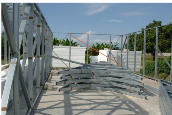
Figure 6.33. Construction of lightweight steel framed house (veerhuis, 2012).
