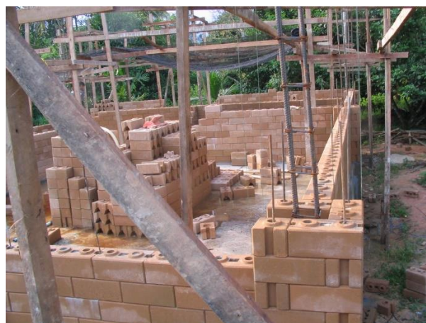
Figure 6.31. Construction of a house with interlocking bricks (Shock Safe Nepal group 1).
