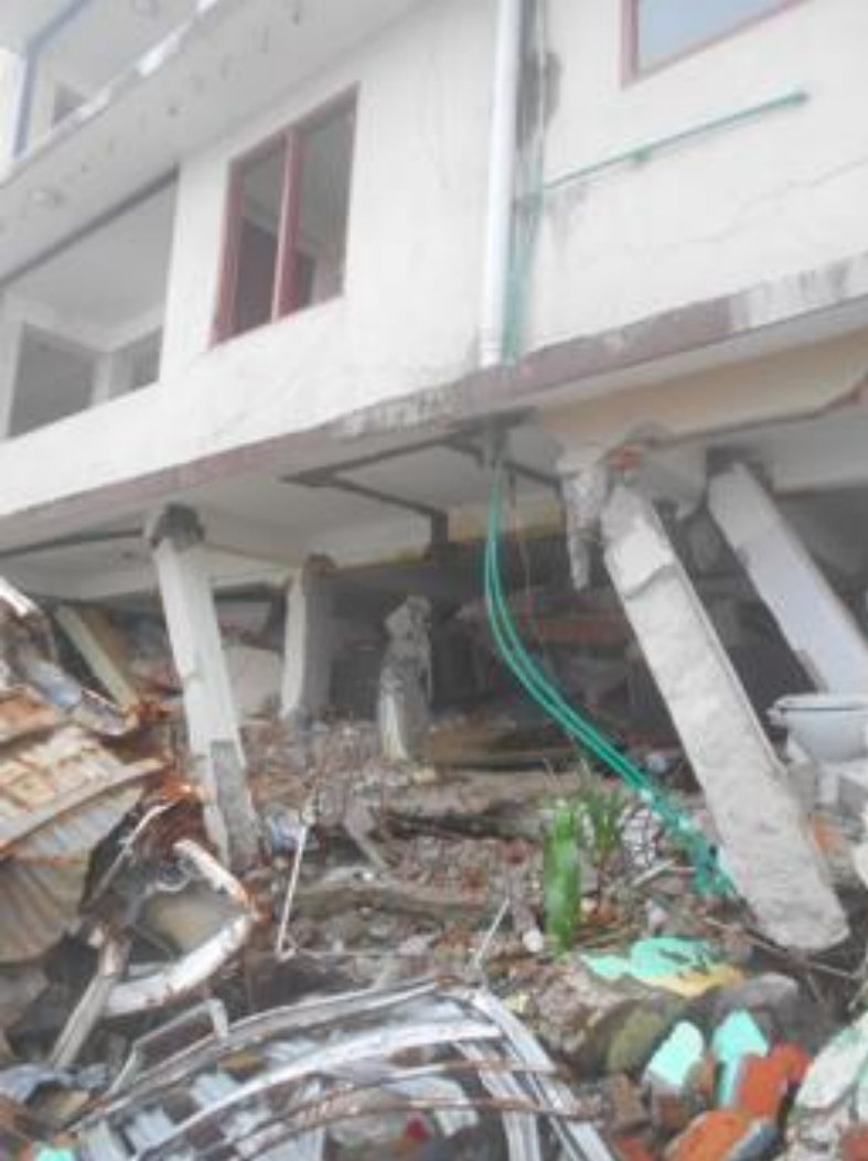
Figure 4.10. Soft storey collapse of RCC-frame building ( Shock Safe Nepal group 1 ).
