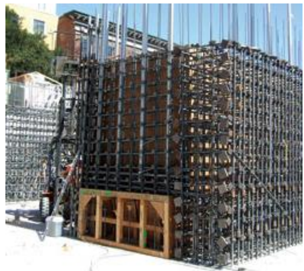
Figure 6.23. Construction of a shearwall (ENR, 2011).
