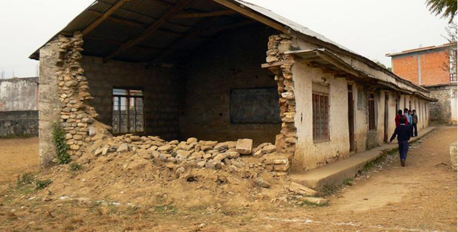
Figure 4.12.: Low strength stone masonry house made with mud mortar (Smart Shelter Foundation).
