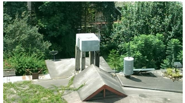
Figure 5.10. Large live loads on roof due to water tanks (Shock Safe Nepal group 1)
