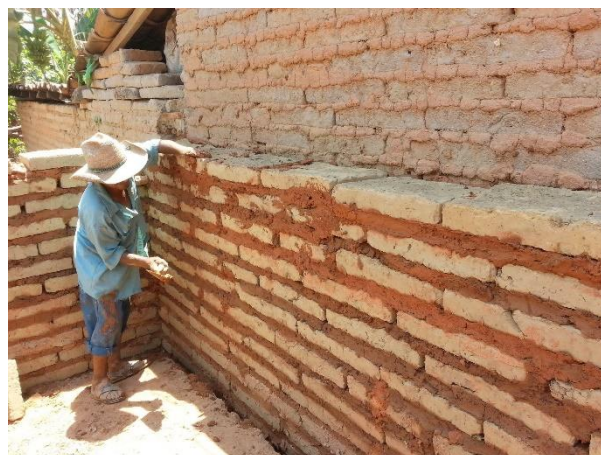
Figure 6.15. Construction of house made with adobe bricks (Municipio, nd.)
