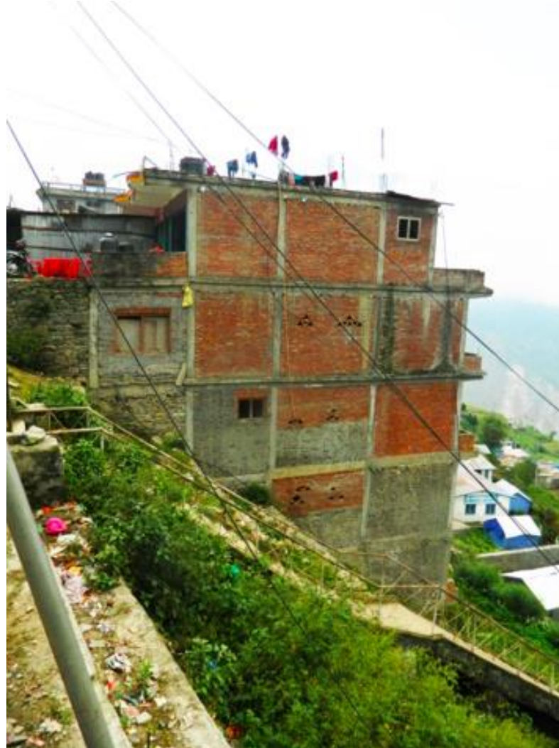
Figure 4.11. Buildings on a slope, discontinuous load path because of construction on the slope ( Shock Safe Nepal group
