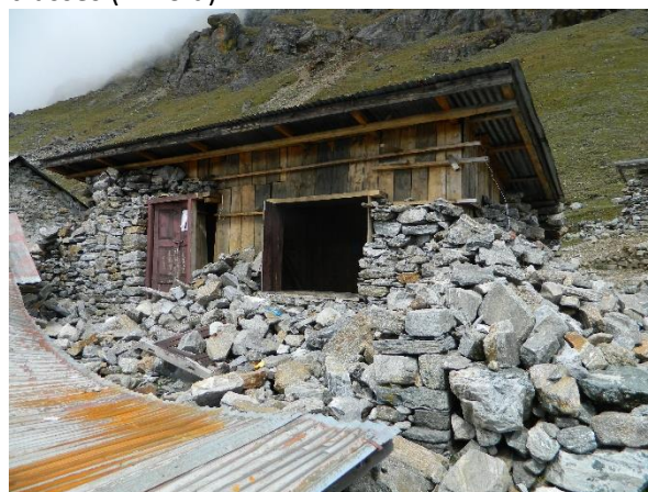
Figure 6.13.: Timber framed house, infill of mountain stone (Shock Safe Nepal group 1).
