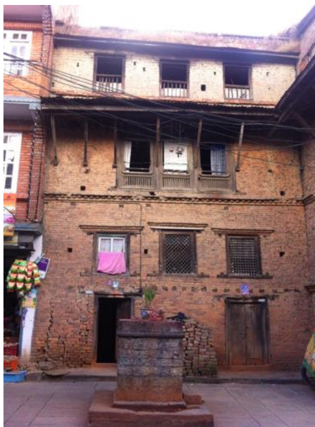
Figure 4.9.: Brick masonry heritage with a newly added floor (Shock Safe Nepal group 1).
