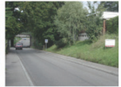
P5 The viaduct with the highway and train-tracks is crossing the residential area of the Eisenbahnweg.
