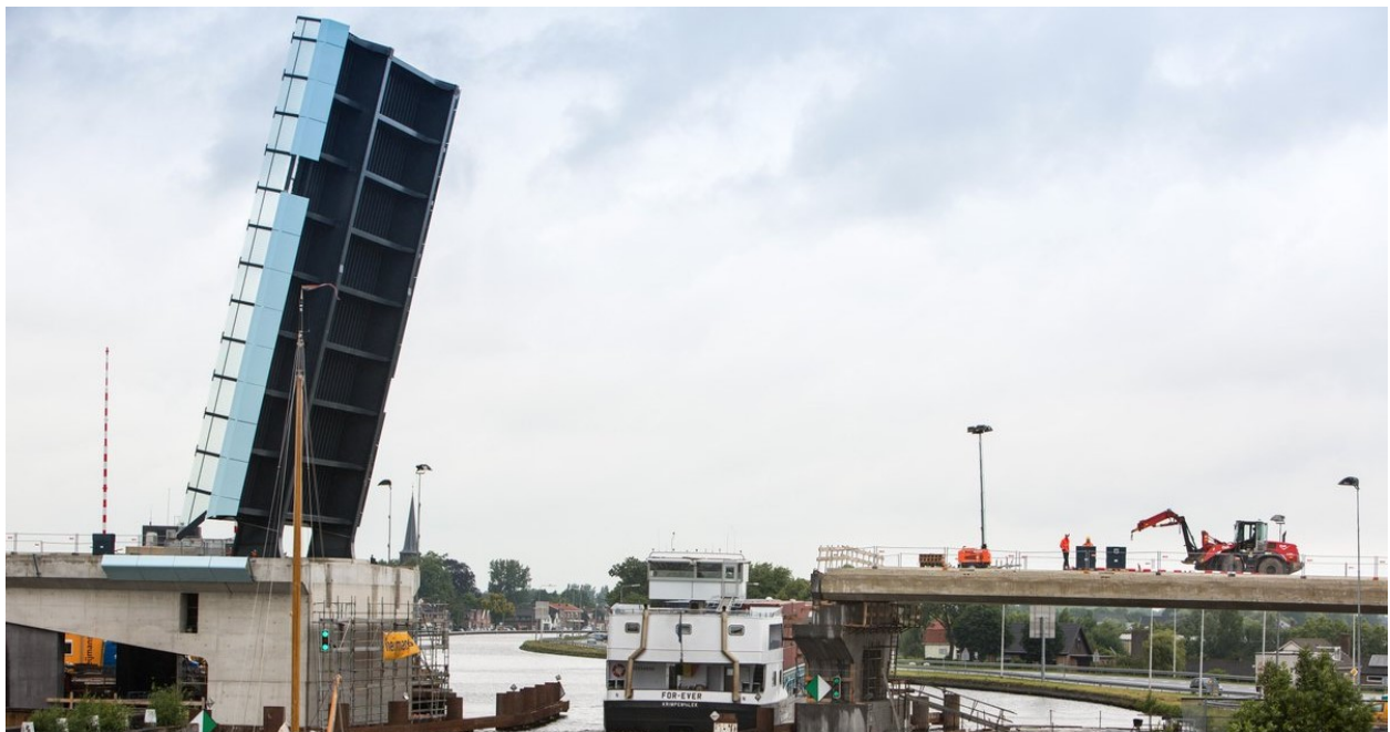
Figure 4-2 Amalia-bridge; picture is taken in the northern direction (Berk, 2016)
