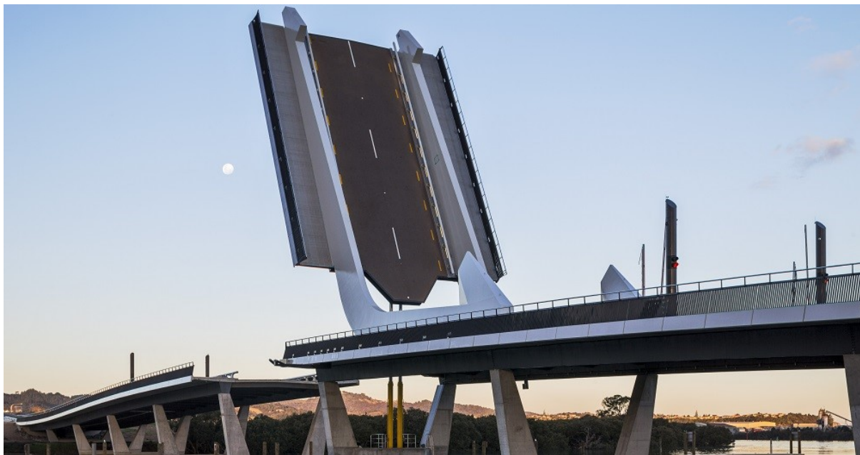
Figure 4-1 Lower Hatea bascule bridge (Reynolds, 2013)
