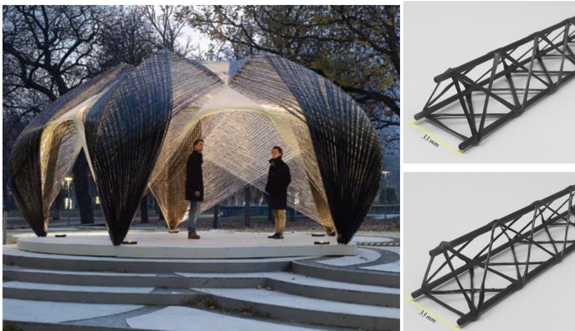
Figure 24: a. Twisted filament wound glass and carbon fiber rovings used in the Research Pavilion 2012 by ICD and ITKE (Knippers, et al., 2015) b. Twisted impregnated carbon fibers as a method to improve the mechanical properties in the WrapTor truss (Woods, 2019)
