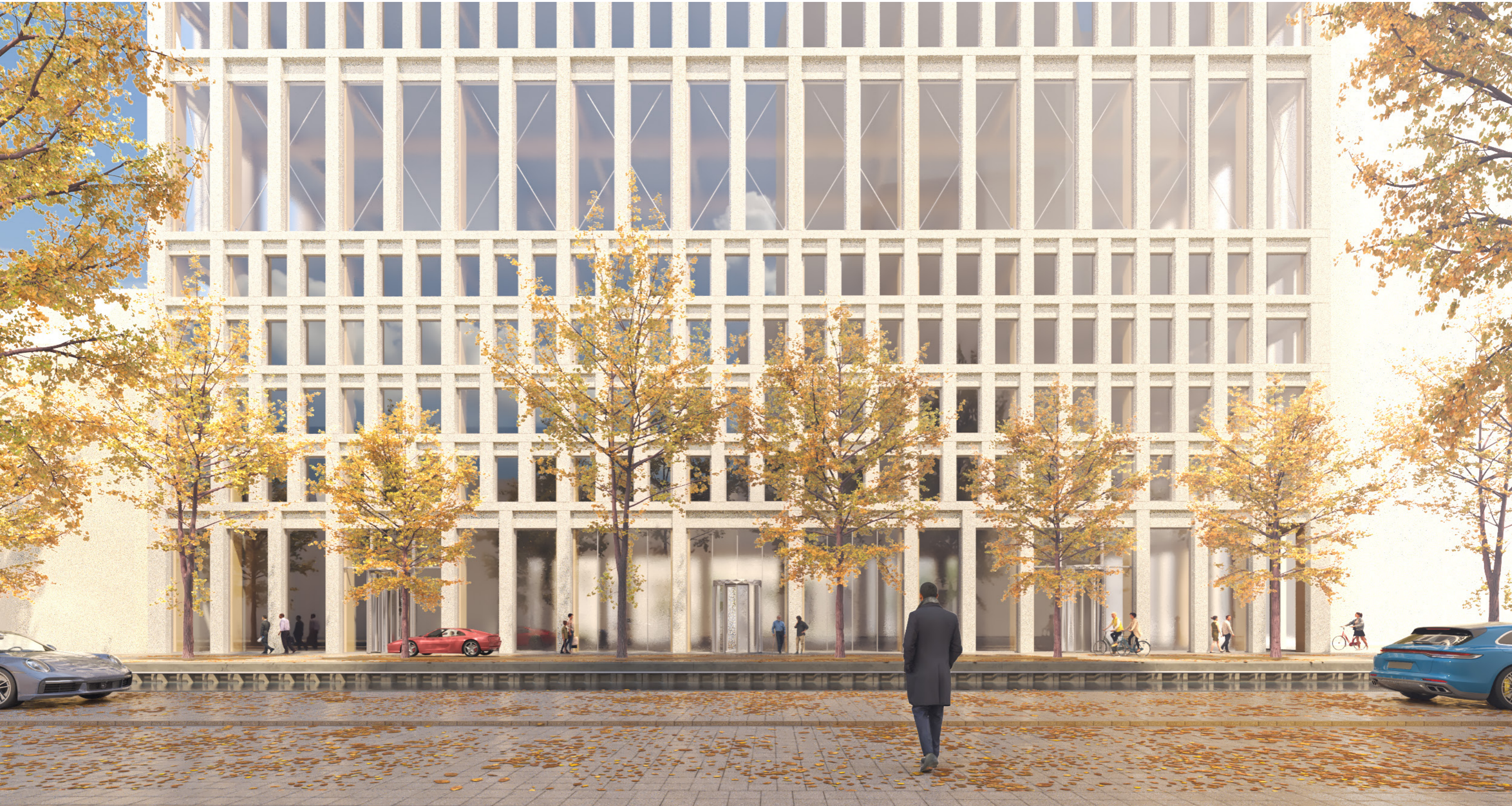
View from Zwarteweg, looking at the entrance of Tower 2 at Oranjevuitensingel
