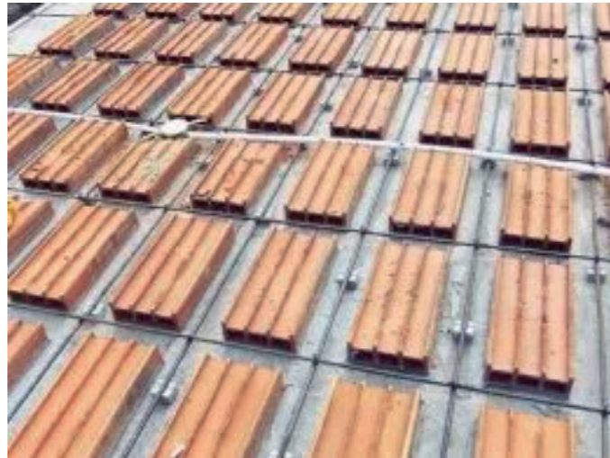
CONCRETE FILLER SLAB
