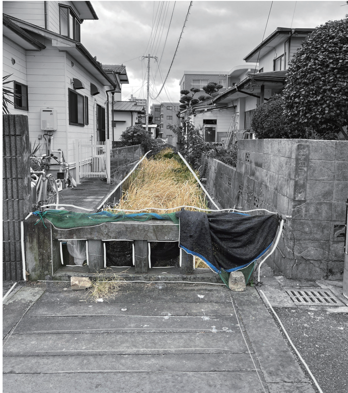
Canal and stone bridge turned into a garbage place
