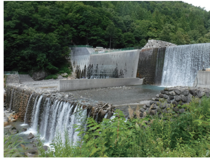
Sabo dam (Hakusan Sabo, 2018)
