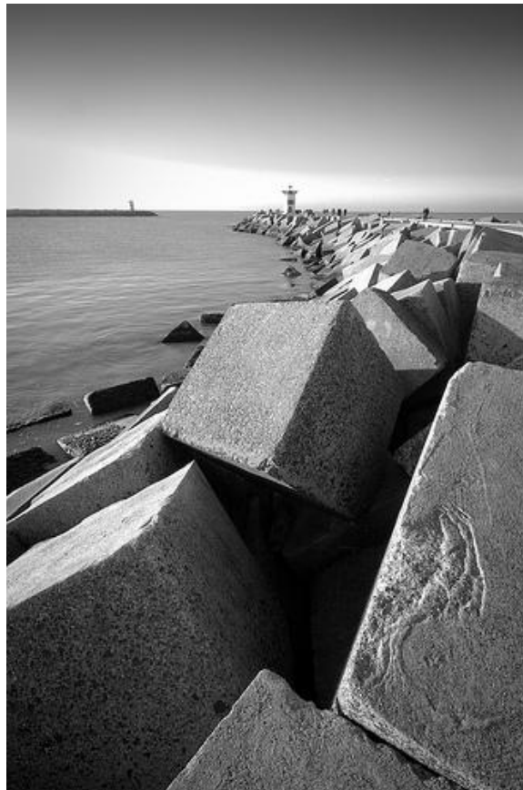
Figure 1. Breakwater with armour layer consisting of concrete cubes
