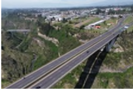
Figure 4. Bridge from Case Study 2
