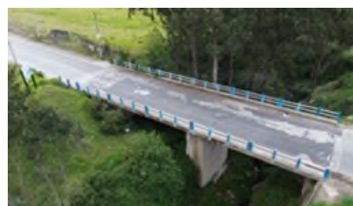
Figure 3. Bridge from Case Study 1
