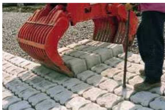
Fig. 4 Placing of Hydroblocks®
