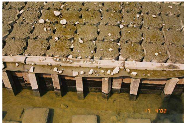
Fig. 12 Detail of a toe construction
