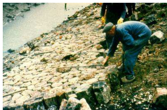
Fig. 2 Pattern placed revetment with natural basaltic columns (Netherlands)
