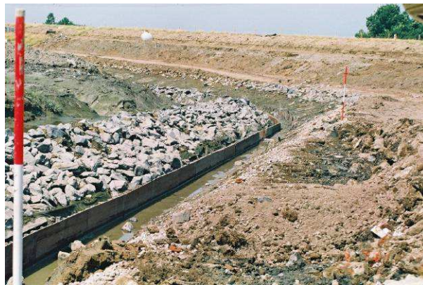
Fig. 13 Toe construction with riprap toe protection
