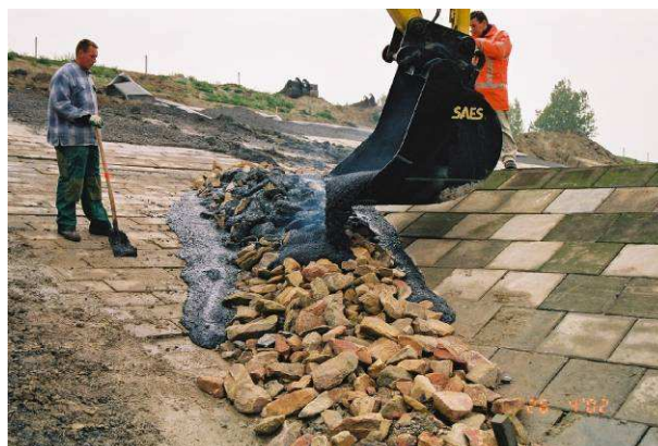
Fig. 18 Transition construction of penetrated rock
