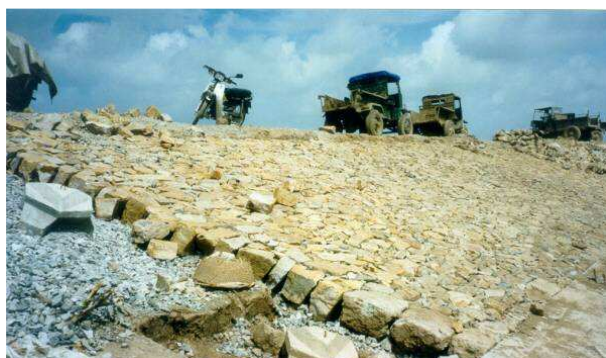
Fig. 1 Pattern placed revetment with shaped natural rock (Vietnam)
