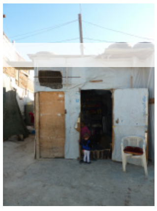
Different construction materials covered with canvas provided by NGO's
