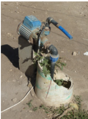
Water pumps are installed, to provide households in water
