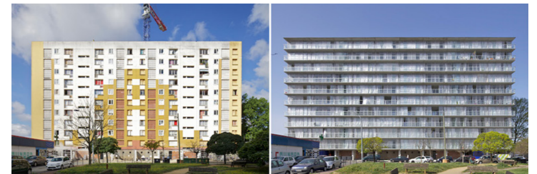
Figure 11: Project 'Transformation of 530 dwellings' shows a non-destructive way for enhancing prefabricated panel construction typologies
