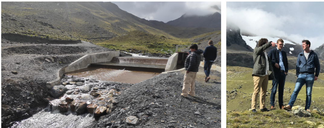
Figure 3.5: Left: Intake structure to divert water from Toma Jumalincu to Pamalarama reservoir. Right: author (left) with H.Kats and supervisor H.G. Nomden, Kaluyo February 2020.
