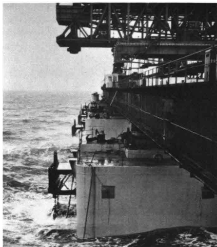
2b Concrete piers on caisson bases sup- port huge shiploader gantry
