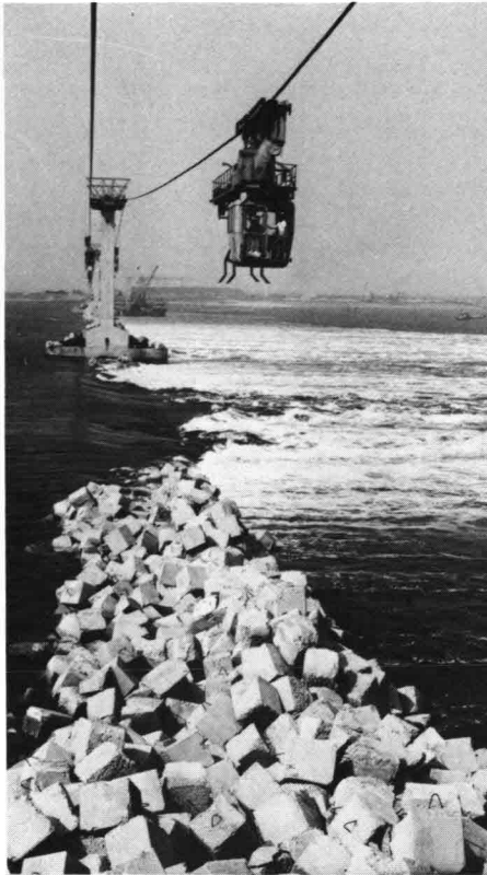
6 Cable railway for dike construction 7 Laying modern, prefabricated erosion protection mattress (Dos I) 8 Erosion protection with asphalt (Jan Heijmans)
