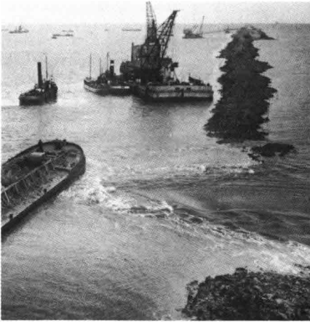
4a Dikebuilding: the both dam sections are approaching
