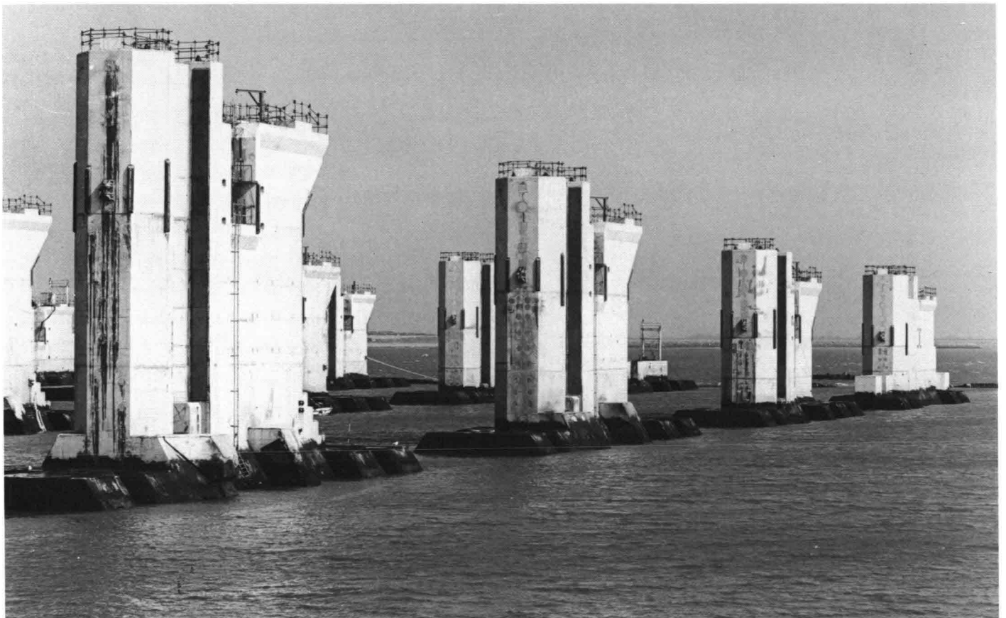
20 First prefabrication dry dock flooded
