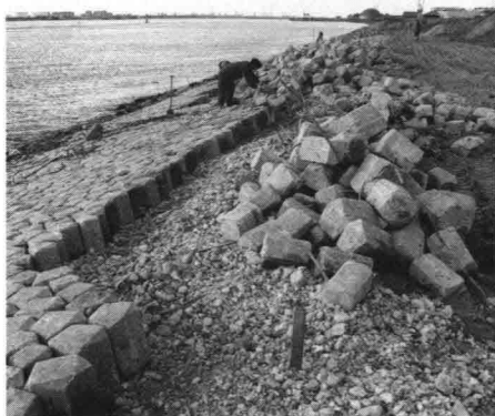
6 Outer berm of a dike protected by polygone concrete blocks
