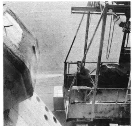
15 Protection of pier by gunnite layer
