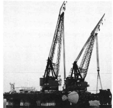
4 Modern offshore construction crane
