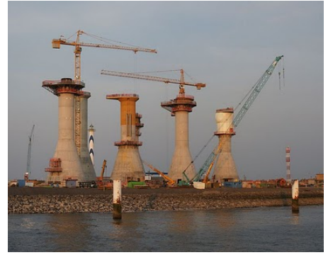
(b) Construction of GBS substructures for Thornton Bank OWF [17]
