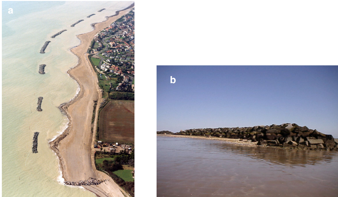
Figure 4 – Elmer defence scheme. a) aerial view, showing tombolo formation on the landward side; b) close up on one structure.
