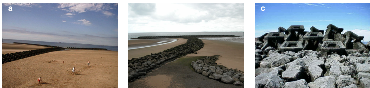
Figure 1 – King-s parade breakwaters in the North Wirral coast (Liverpool): a) Y shaped LCS; b) T shaped LCS; c) close-up of the LCS showing the mixed structure in concrete and limestone blocks.
