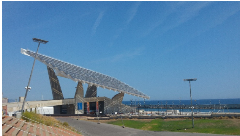
Figure 17 Photovoltaic Installation in Barcelona Port
