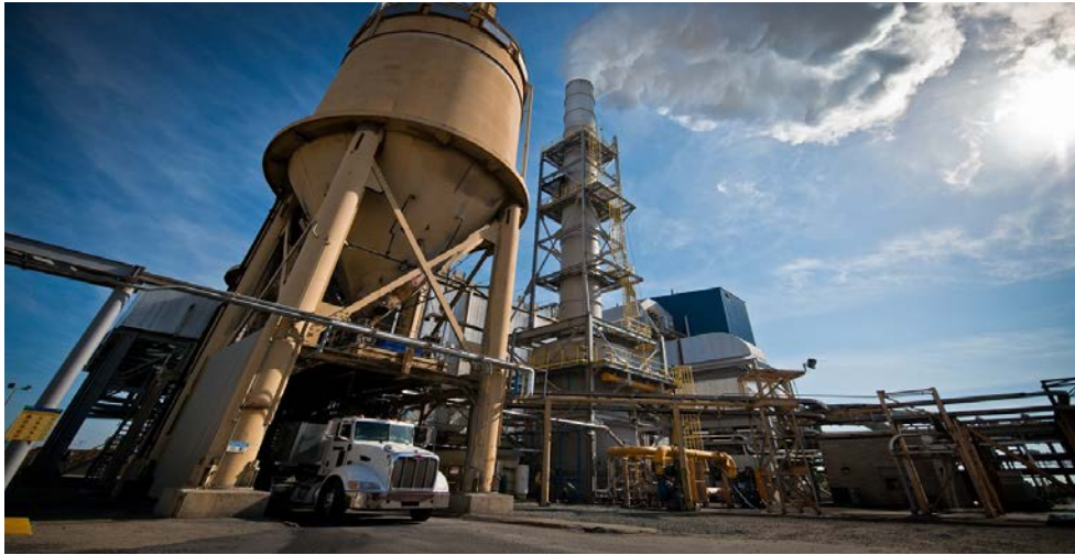
Figure 24 Biomass power plant in port of Stockton, USA (DTE Energy, 2016)
