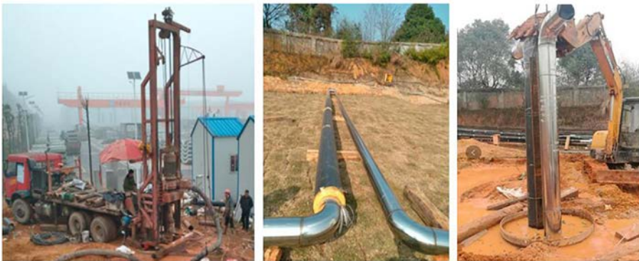
Fig. 12 The schematic diagrams and construction pictures of the vertical UDS system. Reprinted from Z. Liu, Z. Yu, T. Yang, L. Roccamena, P. Sun, S. Li, et al., Numerical modeling and parametric study of a vertical earth-to-air heat exchanger system, Energy 172 (2019) 220–231. Copyright with permission from Elsevier.
