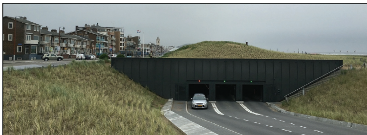
Fig. 3 Photo showing the Katwijk aan Zee seaside boulevard and the entrance to the parking garage under the dunes. (Photo by J. Figlus.)
