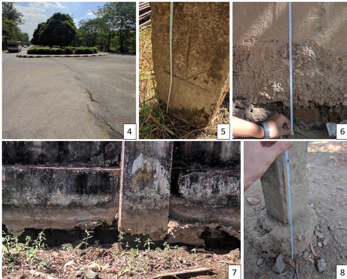
Fig. 6.5: Visuals on possible effects of subsidence. Picture four shows differential surface motion in a road. In picture five, a level is indicated which might show a previous surface level. Pictures six and seven show parts of structures that are revealing because of a lower surrounding surface. Picture eight shows a possible effect of surface erosion. The locations of each picture are shown in Fig. 6.3. Source: Boy-Santhos van der Sterre
