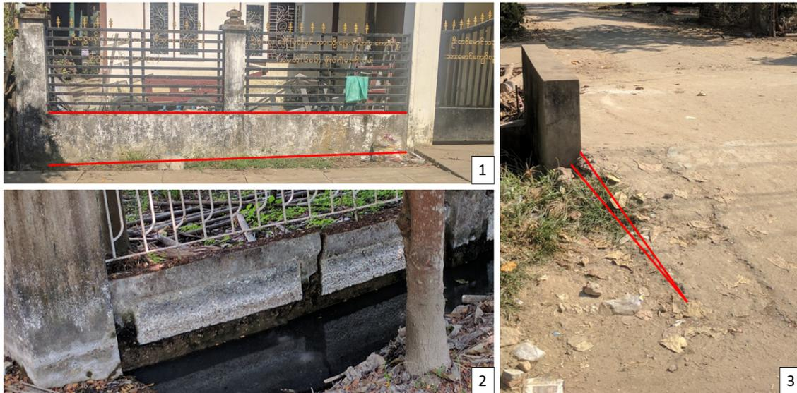
Fig. 6.4: Visuals on possible effects of subsidence. Picture one and three show sloped terrain near a possibly founded structure. In case of subsidence, the structures remain in place while the surrounding areas gradually go down. Picture two shows damage that may result from differential surface motion. The locations of each picture are shown in Fig. 6.3. Source: Boy-Santhos van der Sterre
