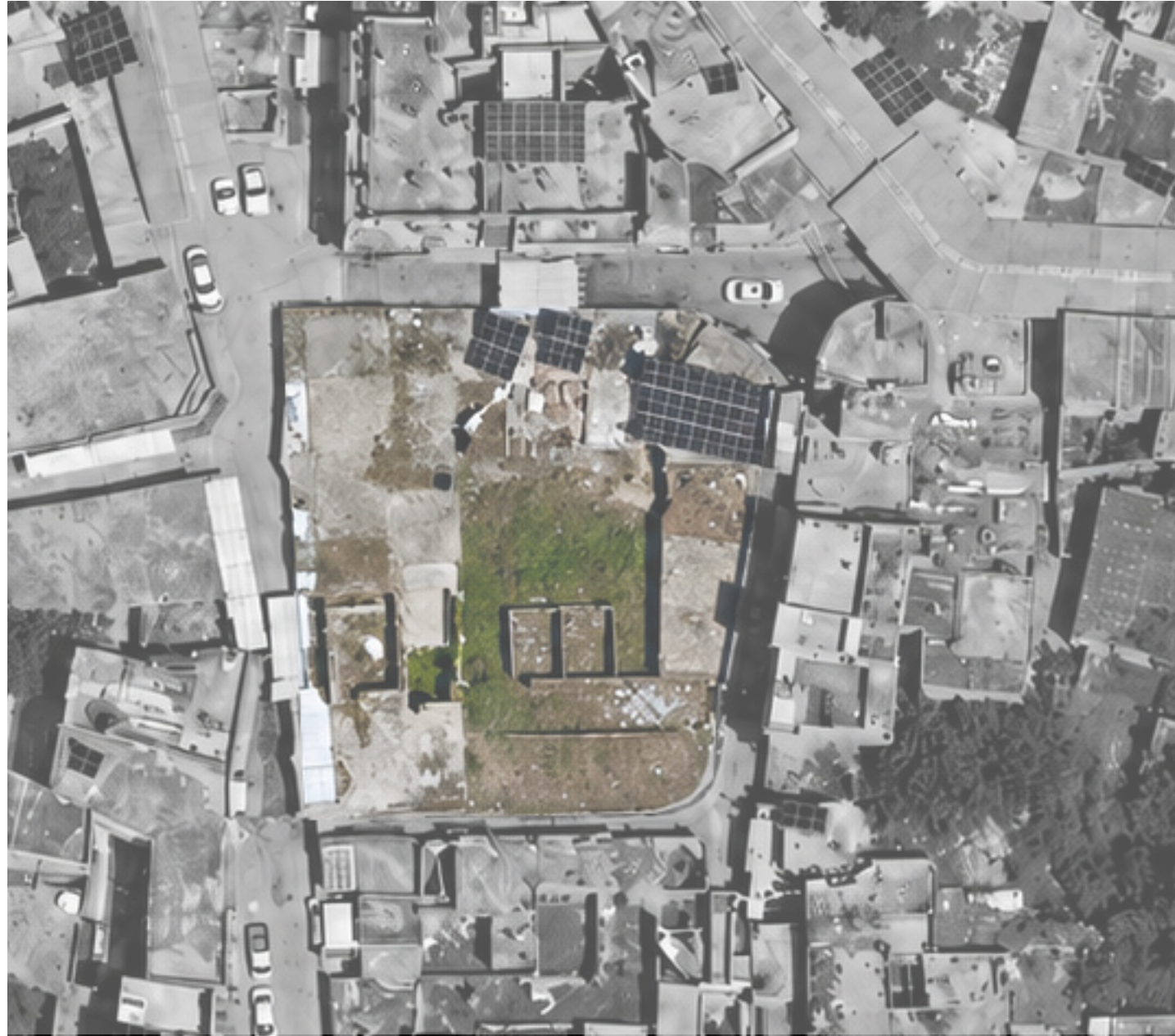
Figure 3 | Pre-Existing Structure before the development.
