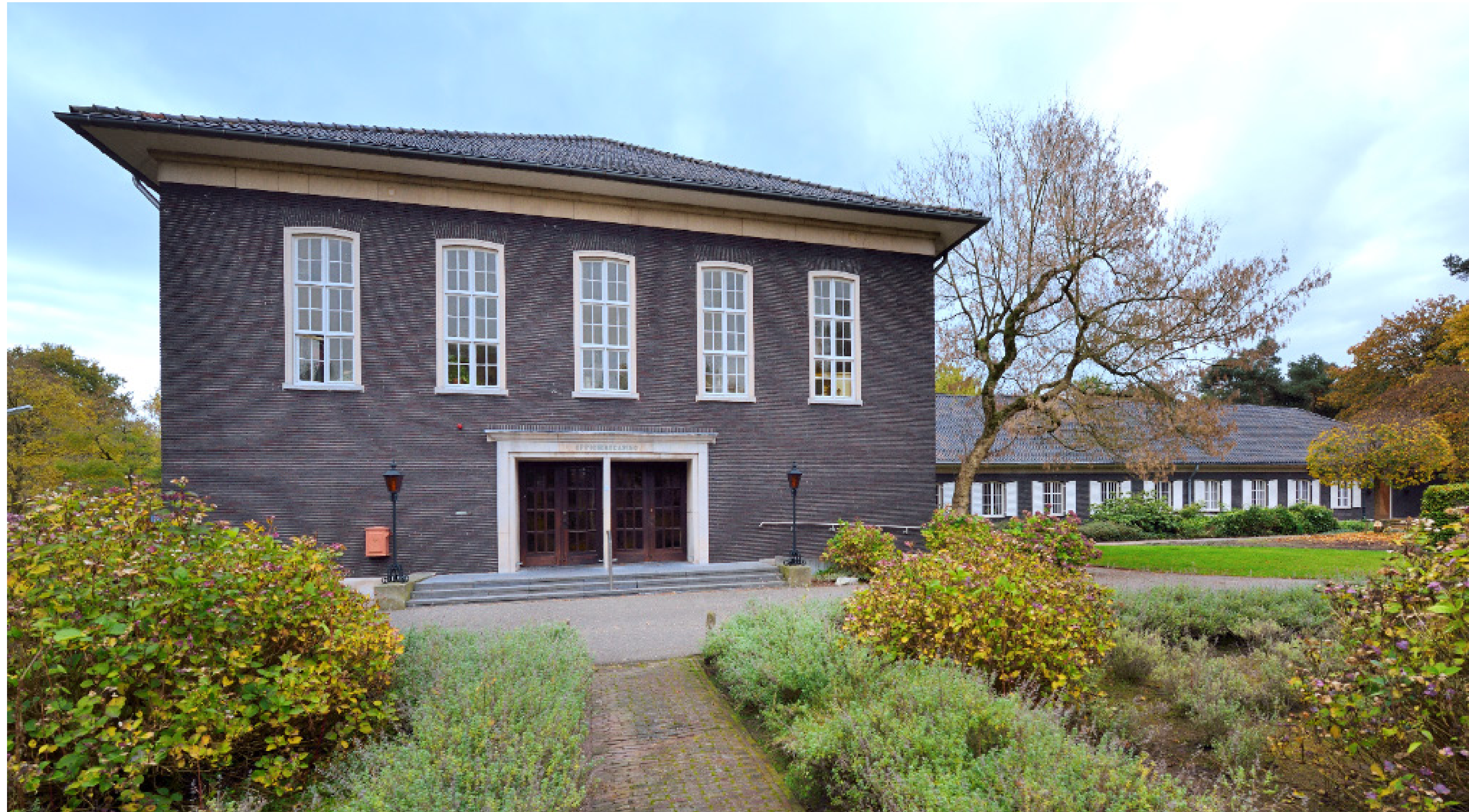
Source: Current photo of front facade. (Officierscasino: Toelichting, n.d.)
