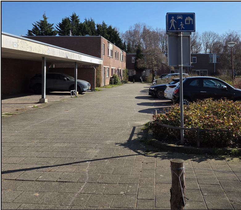
Figure 25: picture of current site showing that the woonerf is designed for car-mobility rather than human daily use, which results in a lot of pavement
