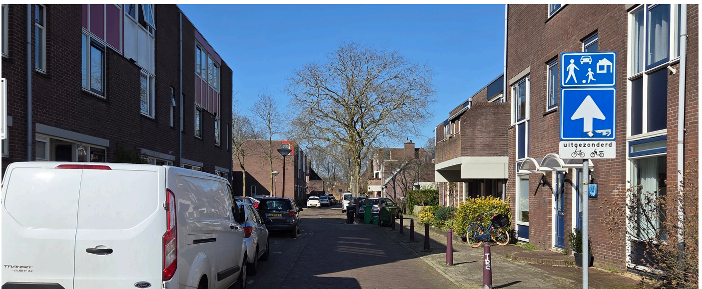
Figure 18: A street type woonerf showing the importance of thresholds between infrastructure & movement (source: author, 2025)
