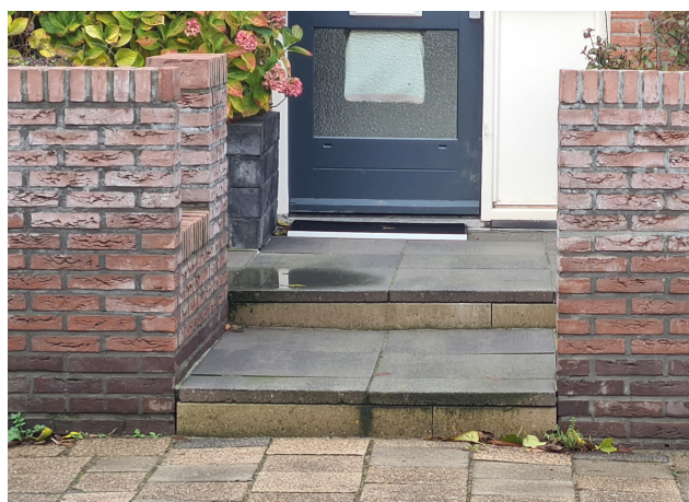
Figure 10: Raised threshold seems fine, but makes it less accessible for people who are less mobile (photograph by author, 2025).
