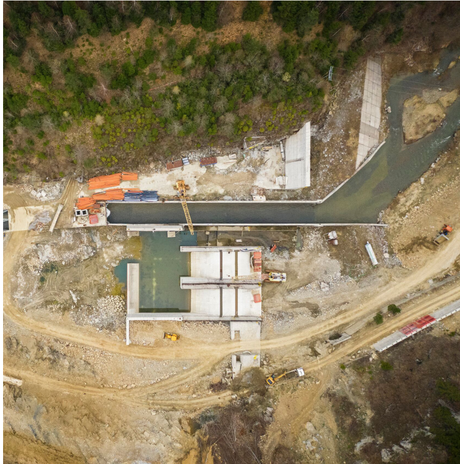
Figure 15: One of the building sites visited during field research in Romania
