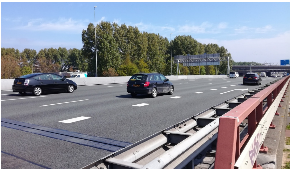
Fig 3. A10 Highway – main physical barrier in site
