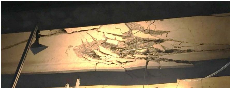
Figure 8 Shear failure beam test 1
