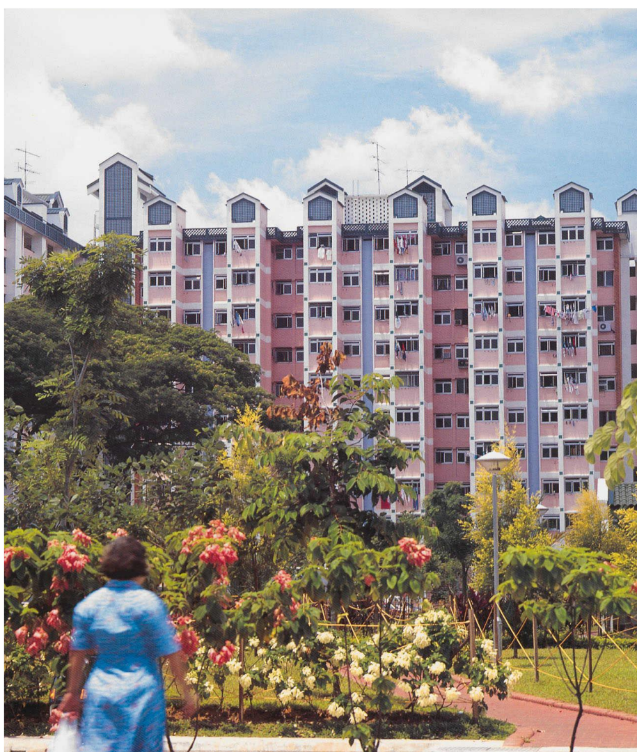
(Fig. 3) Kim Keat Court Demonstration Phase upgrading project, c.1995. HDB Annual Report 1994-95 (Housing & Development Board, 1995). Collection of the National Library Board Singapore.
