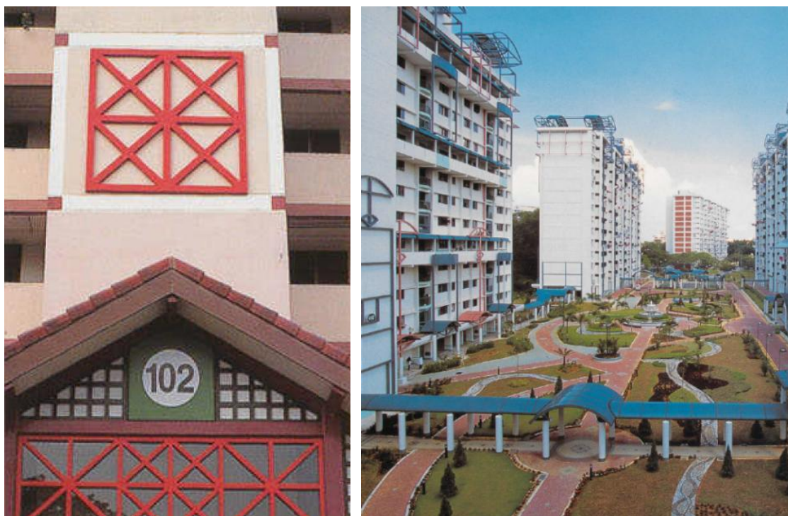
(Fig. 16) Decorative features at the Crescent View upgraded precinct, c.1998. HDB Annual Report 1997-98 (Housing & Development Board, 1998). Collection of the National Library Board Singapore.
