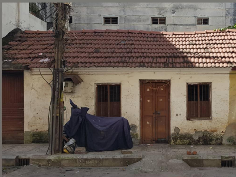
An old residential building.
