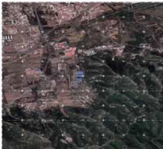
Type F Buildings along/ in mountains
