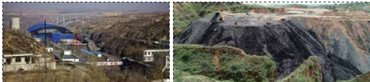
Fig.2.20 The Jiaoyao coal mine factory in Handan was the best representative of the development of local small industrial enterprises in China in the 1970s. Source: https://m.fang.com/news/yz/0_9520395.html http://www.hynews.net/dxb/dysqxb/07/1207/20/3V4V20A0000120GU.html
