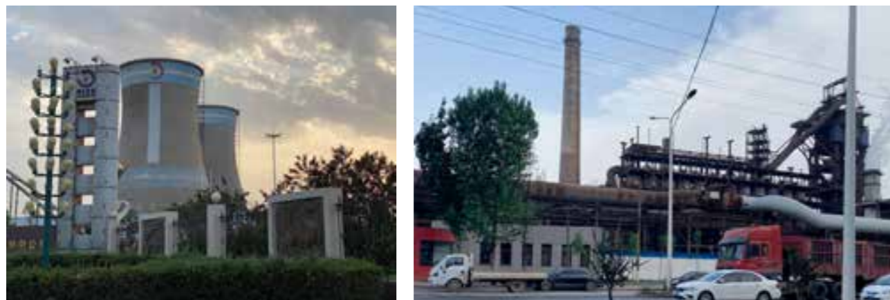
Fig. 6.1.1 Industrial buildings, structures, and other construction space Source: author
