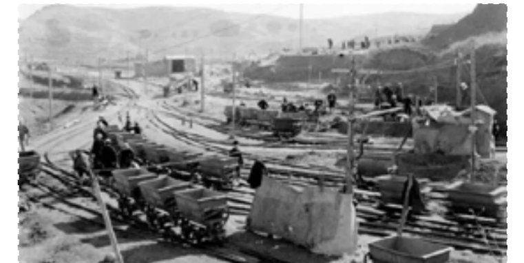
Fig. 4.3 Industrial belt construction https://www.sohu.com/a/340272423_750659
