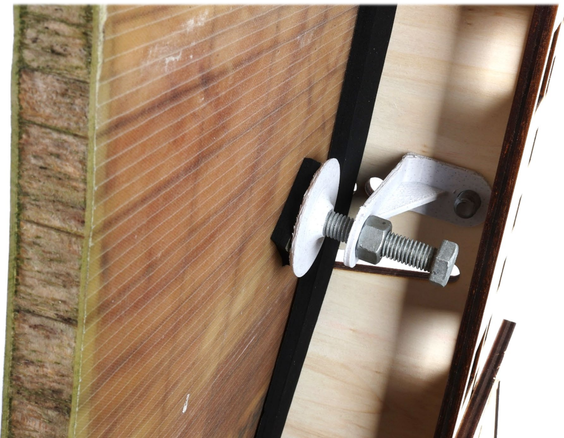
Figure 89: Final iteration of the adjustable clamp with compriband for acoustic sealing
