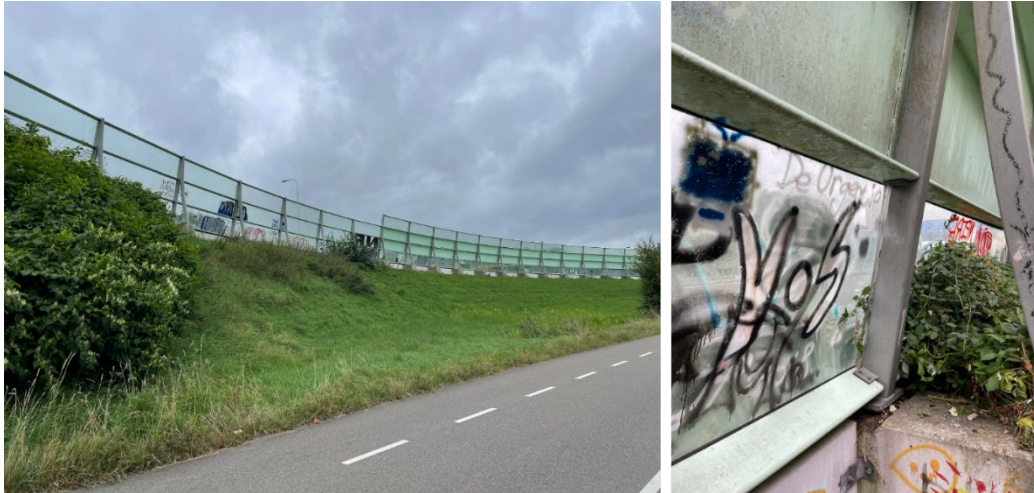
Figure 25: A reflective, tilted barrier made of glass and uses a triangular frame.
