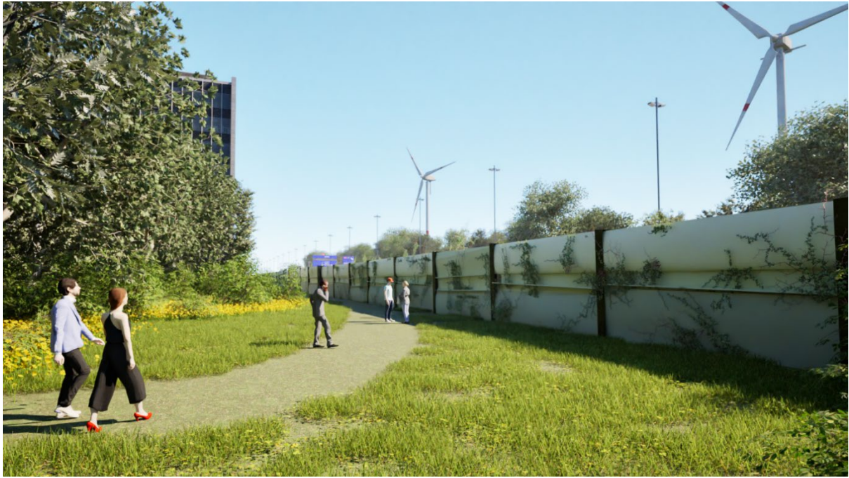
Figure 98: Perspective of the residents or landscape users, showing the back of the noise barrier design with climbing plants and alternatively oriented panels.
