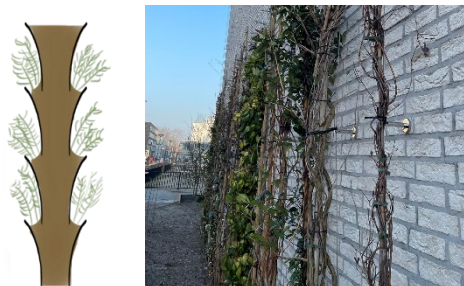
Figure 49: Vegetation options for this concept. A) soil in between panel rows. B) wire structure with spacers.
