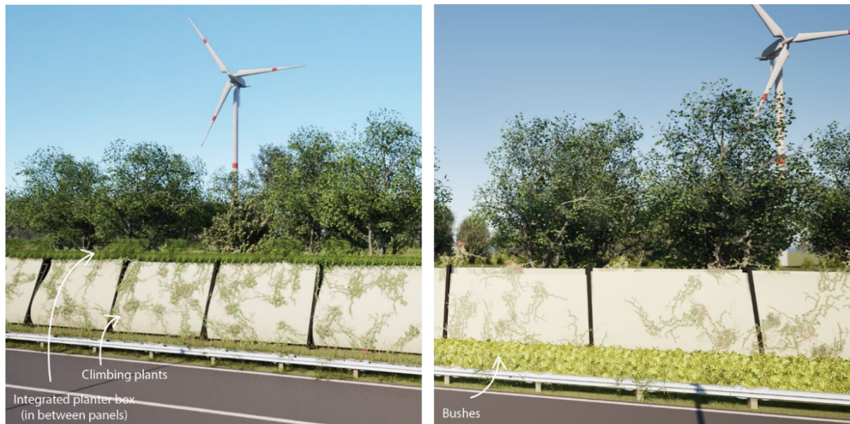
Figure 92: The noise barrier design in a rural environment, with three vegetation options: climbing plants, integrated planter box and vegetation around the barrier. This can also be done on the resident side.
