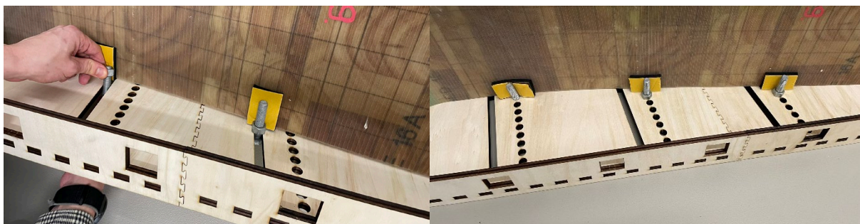
Figure 123: Slotted bolt (left) and perforated bolts in the connection points along the height of the cassette. Rubbers are placed between the bolt / nut combination and the panel.
