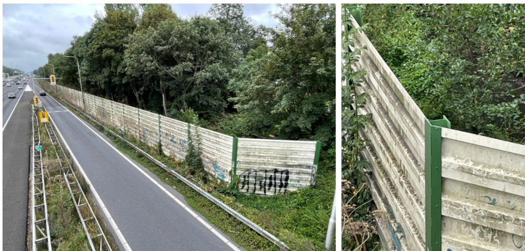
Figure 26: A white corrugated metal sheet placed in between H-beams.
