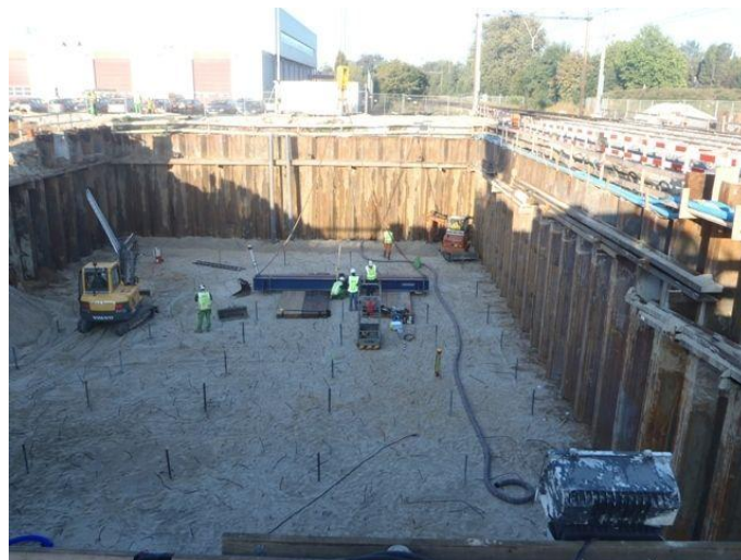
Figure 10.7: Excavated cofferdam made of pile sheets [52]
