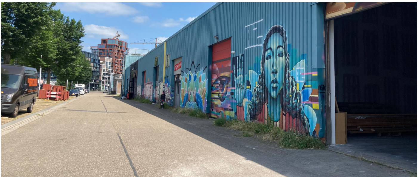
Figure 115: Existing business spaces for businesses light industry activities in NDSM-Werf Oost [Own photograph]
