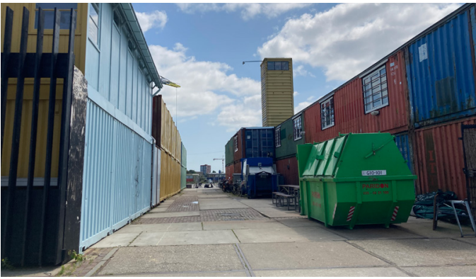
Figure 109: Temporary workspaces in NDSM-Werf Oost [Own photograph]
