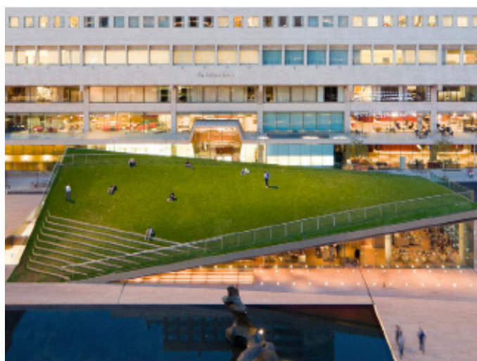
Figure 82: Reference image for sloped green roof building (retrieved from Gemeente Amsterdam, 2020a).
