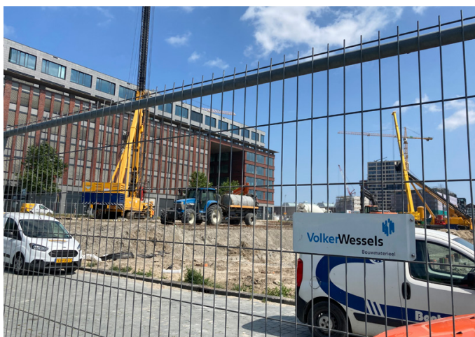
Figure 93: Block B10 under land preparation [Own photograph]
