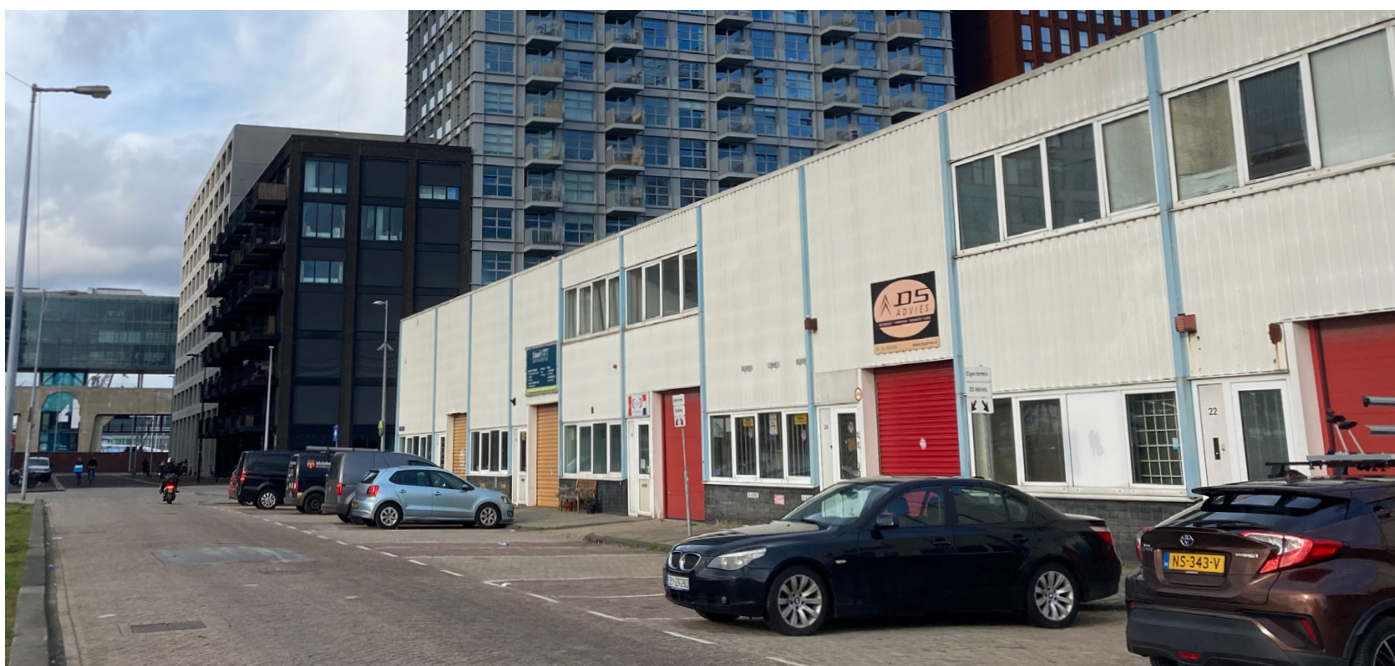
Figure 57: A range of existing businesses identified as light industry in NDSM-Werf West (A-blocks) [Own photograph]
