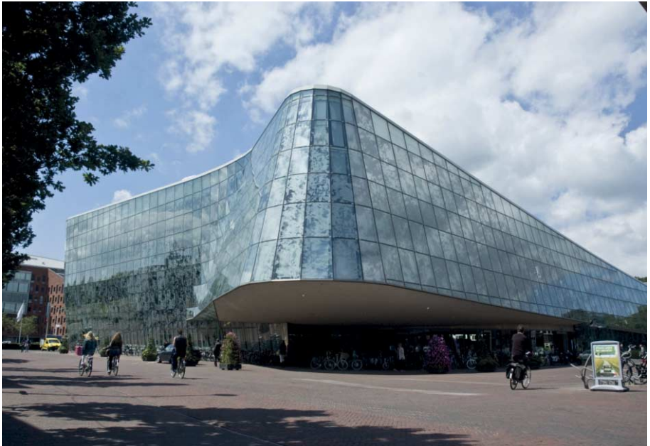
FIG. 229 The front façade after completion
