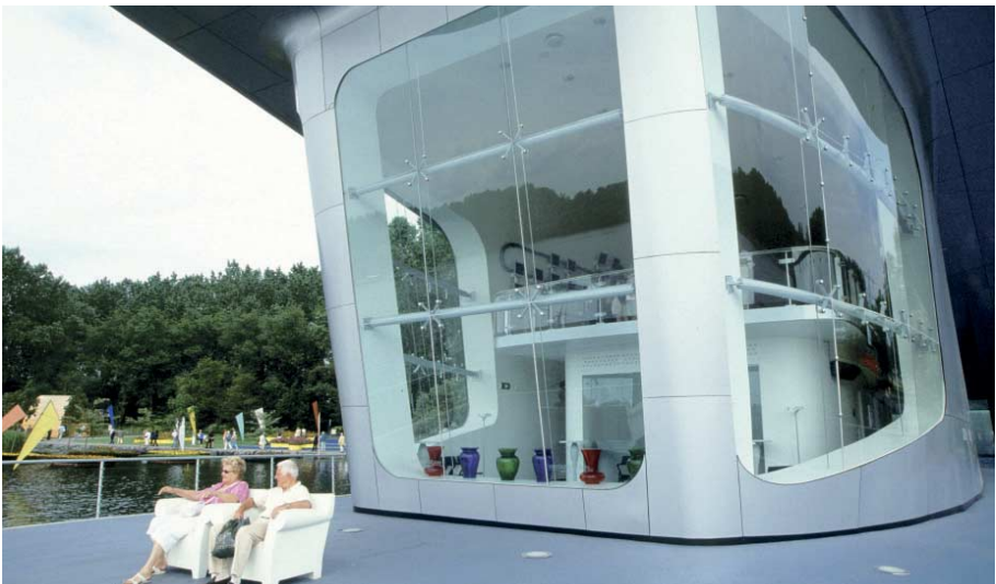
FIG. 194 Exterior view of the southern façade
