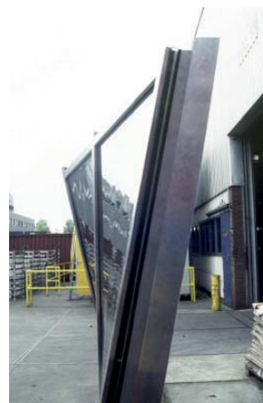
FIG. 100 Mock-up of a twisted façade as developed with Reynolds
