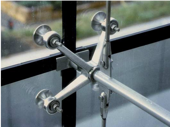
FIG. 80 Details of glued connection and spider web arrangement
