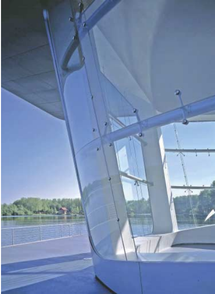
FIG. 192 Southern façade with curved glass panels.
