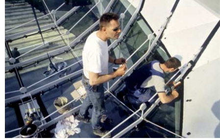
FIG. 189 Assembly of the ode-shaped suspensions
