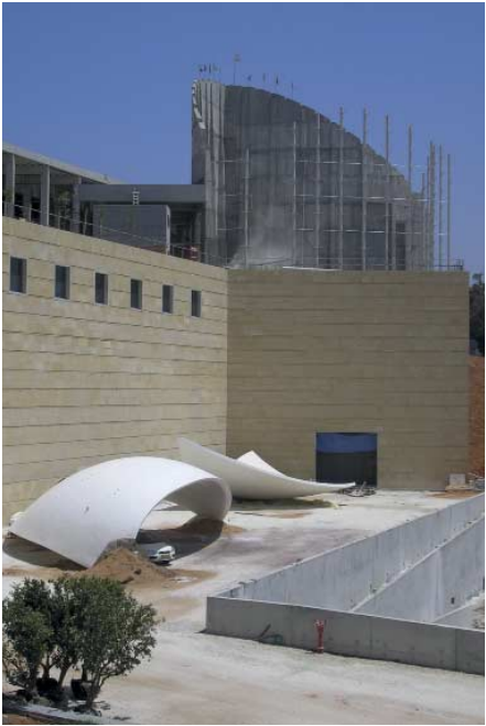
FIG. 154 Preparation and hoisting of the upper and lower wing of the Library in August 2005
