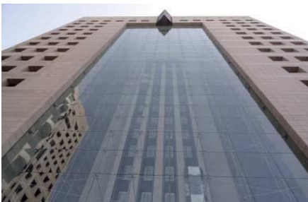
FIG. 260 View of the frameless glass façade of the OZ building
