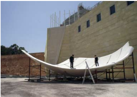
FIG. 156 Bolting glass fibre polyester plates on the seams before applying the finishing layer
