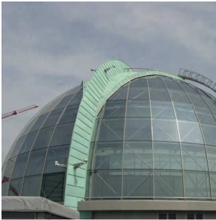
FIG. 175 Exterior of the dome, the insulated glass-panels and their transparency towards the interior of the dome
