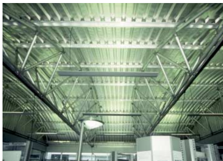
FIG. 207 Space frame in the Aluminium Centre
