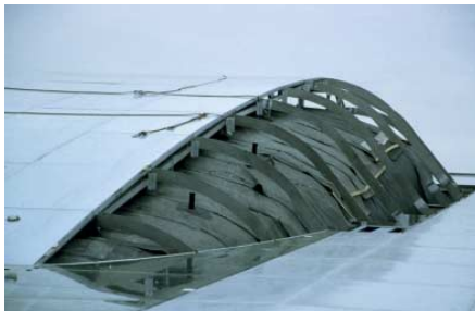
FIG. 186 Opening for the bent panels
