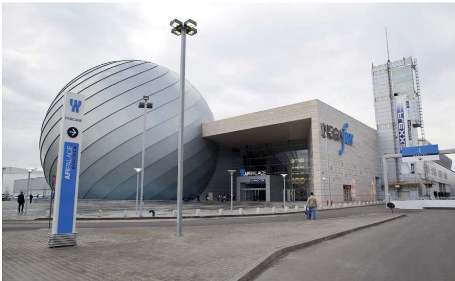
FIG. 262 View of the 42 m diameter sphere, built up as a steel structure, aluminium battens, timber planking and zinc cladding as the covering of the IMAX theatre
