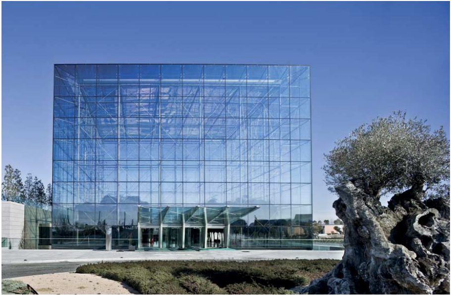
FIG. 257 Outside view of the Glass Cube Santander Bank, Madrid
