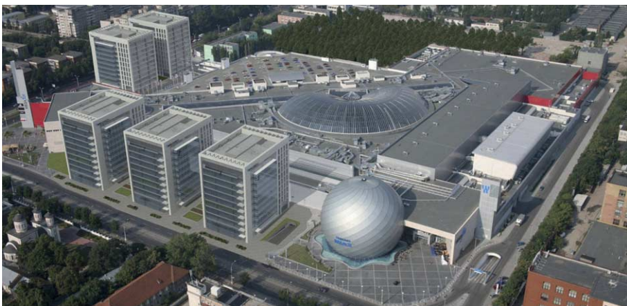
FIG. 274 Overview of the total complex
