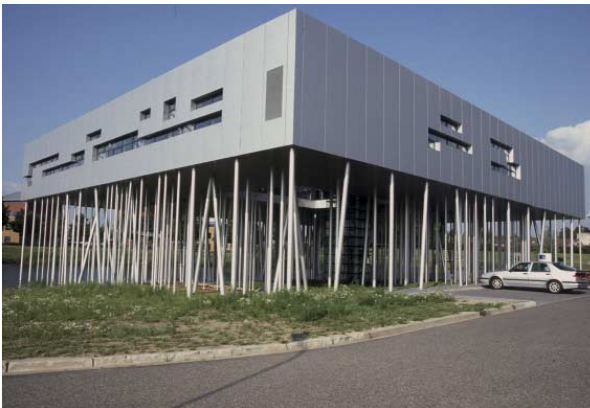
FIG. 204 Exterior of the Aluminium Centre
