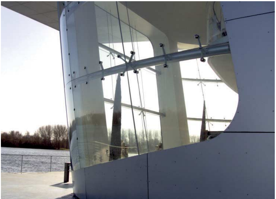
FIG. 106 Cold bent glass laminated panels in the Floriade building Haarlemmermeer
