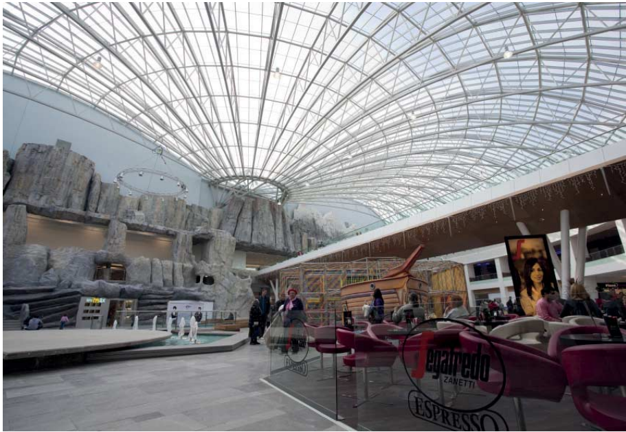
FIG. 272 Dome after completion
