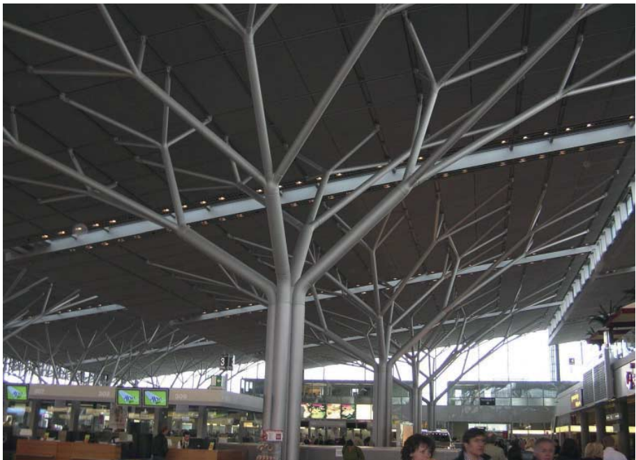
FIG. 37 Passenger Terminal, Stuttgart
