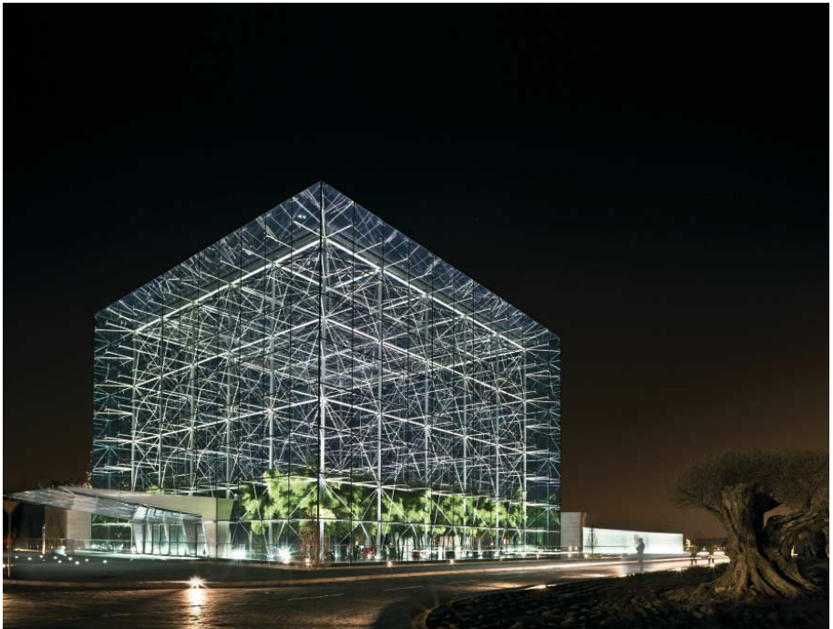
FIG. 258 Outside view of the Glass Cube Santander Bank, Madrid
