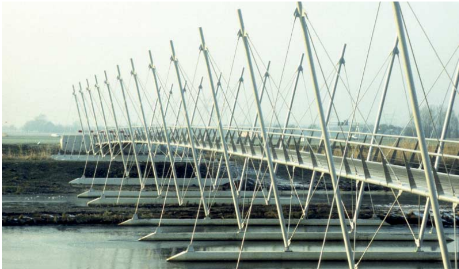
FIG. 196 Tensegrity Bridge in Purmerend
