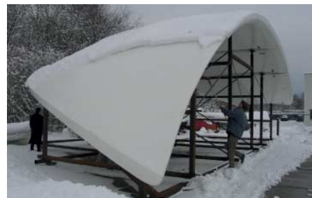
FIG. 151 Fitting of all the roof segments at Lelystad
