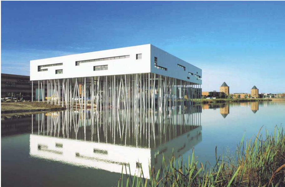
FIG. 213 Exterior of the Aluminium Centre
