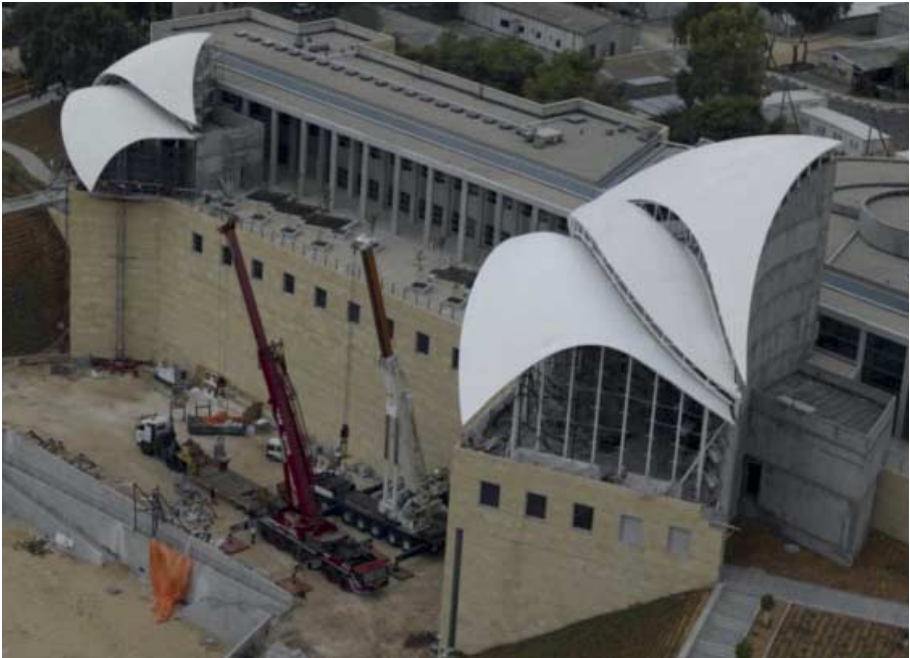
FIG. 157 View of the building site on 6 th of November 2005, photographed by Ardon Bar Hama
