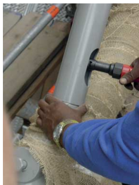
FIG. 171 Installation of a diagonal tube to the horizontal ring nr. 18
