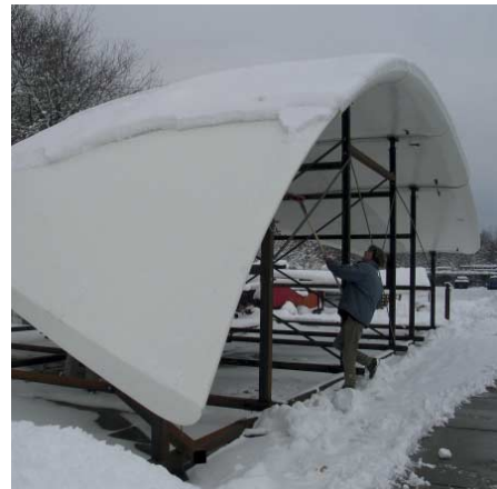
FIG. 61 GRP stressed skin mock-up for the roof
