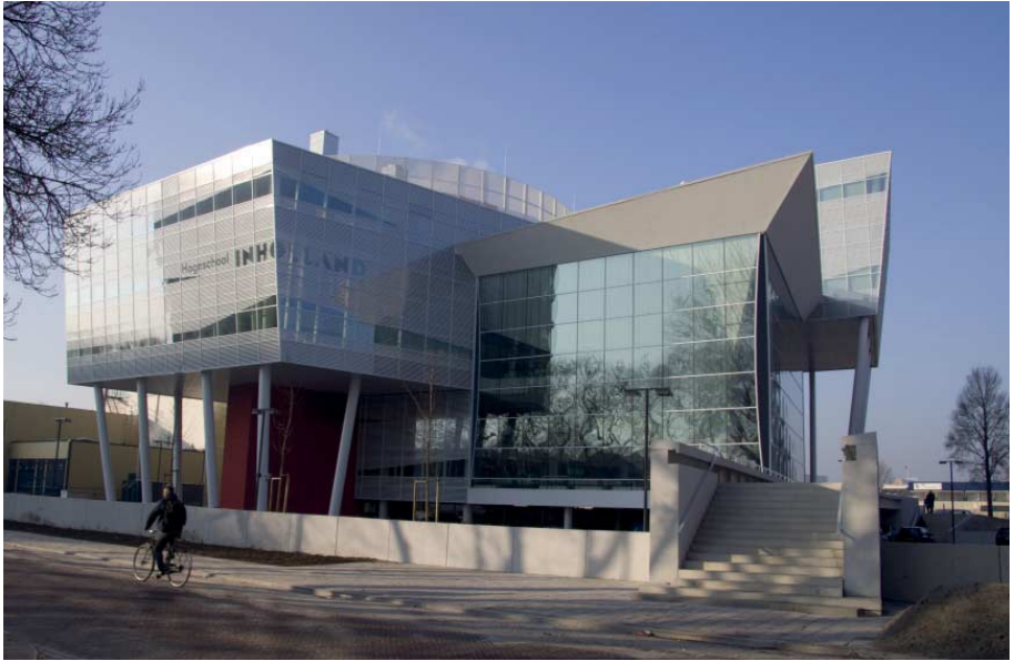
FIG. 286 Overall view of the two large facades. Clearly visible are the two lens-formed rubber corner fillings. The third façade on the right hand side around the corner, only 3 m wide
