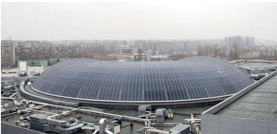
FIG. 273 Overview of the dome
