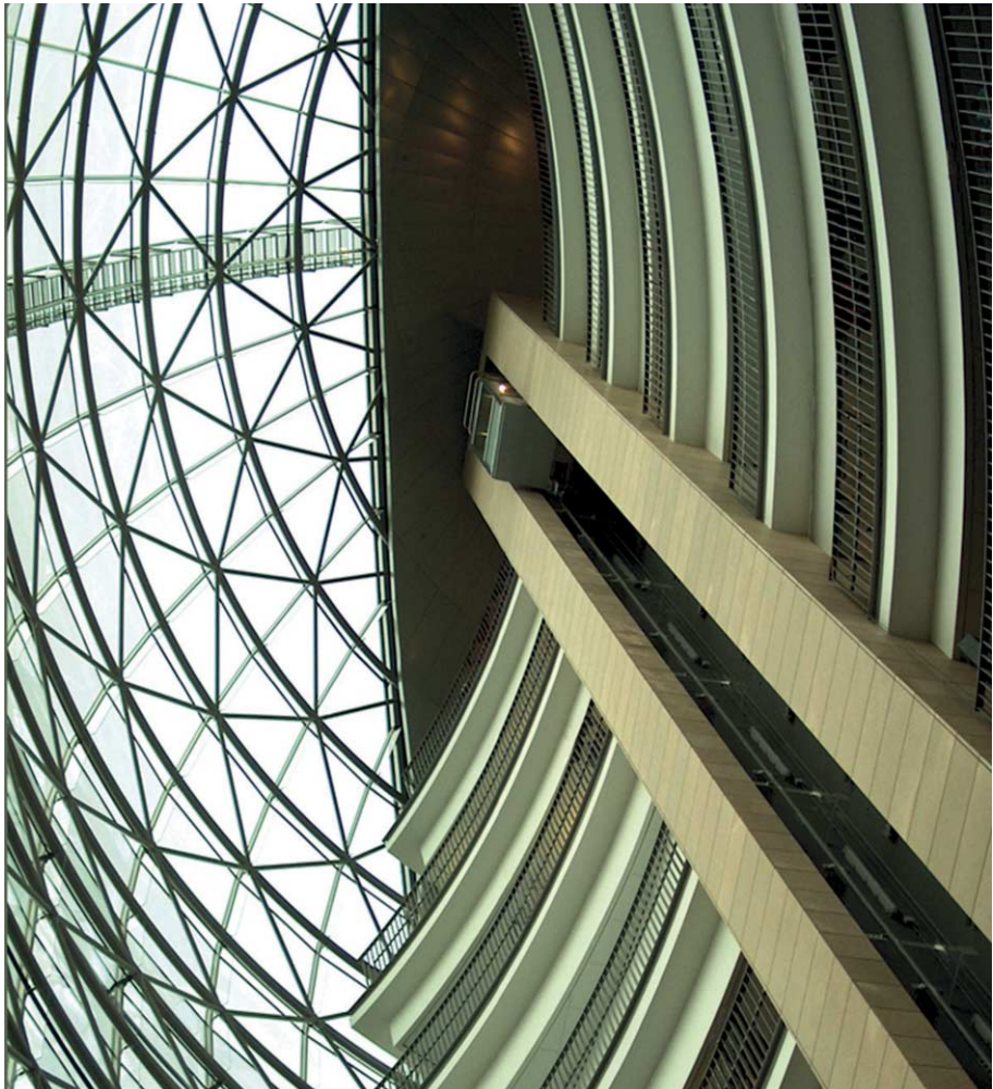
FIG. 167 Looking upward in the atrium void
