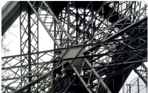
FIG. 20 Details of the 1889 Eiffel Tower composed of wrought iron elements, at the time an old-fashioned material
