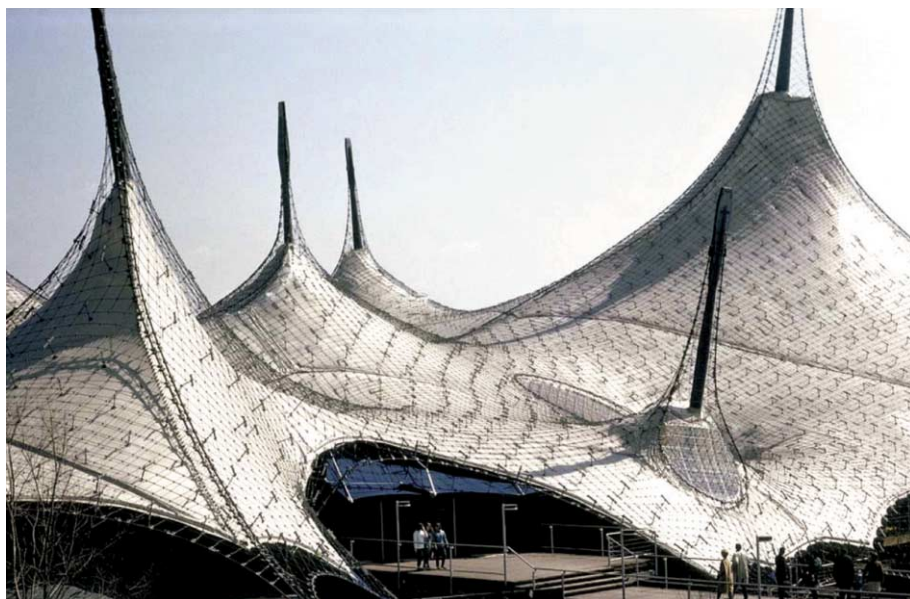
FIG. 06 Olympia Roof in Munich, Frei Otto
