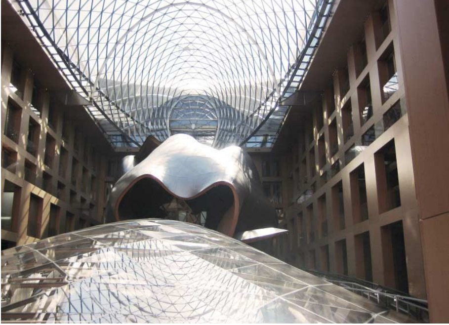
FIG. 219 Interior of the DG Bank in Berlin
