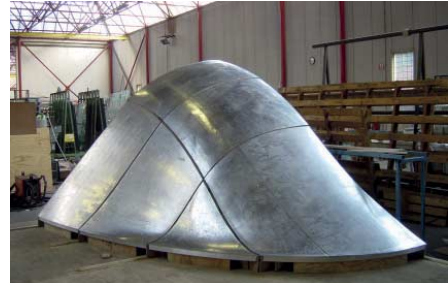
FIG. 185 Completion of all bent panels for one side
