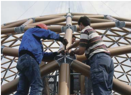
FIG. 118 First time build up of the cardboard dome in IJburg
