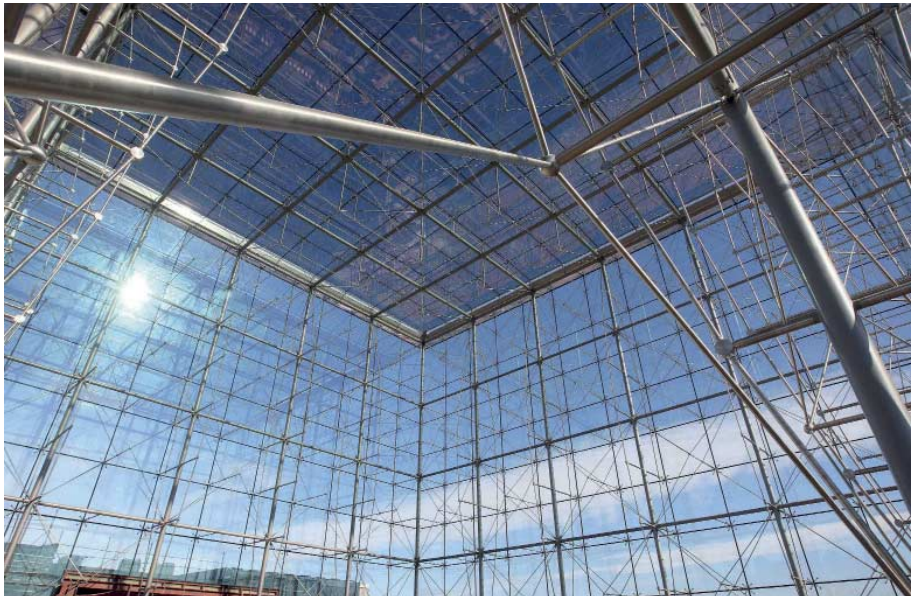
FIG. 256 Inside view of the Glass Cube Santander Bank, Madrid
