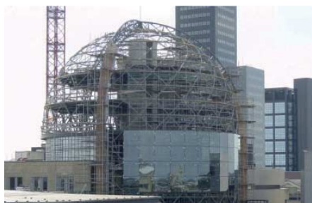
FIG. 165 View of the dome under construction
