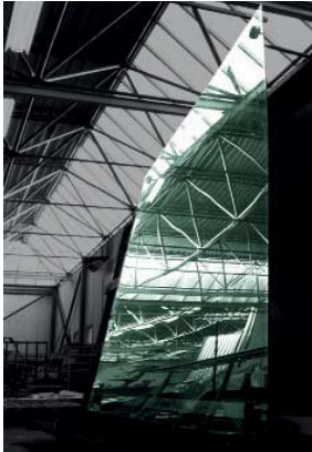
FIG. 103 Cold twisted glass panels
