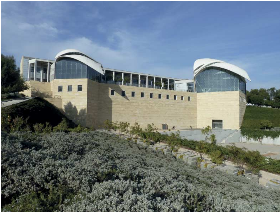
FIG. 158 Overview of the building site after completion
