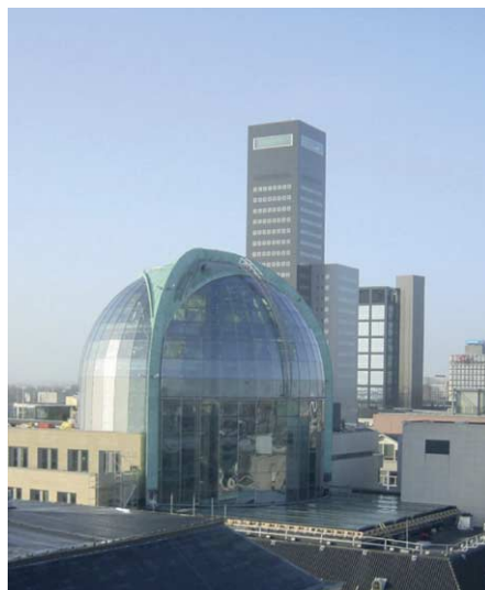
FIG. 179 Northern side of the dome with the lower roof. In the back the 114 metre high Achmea tower
