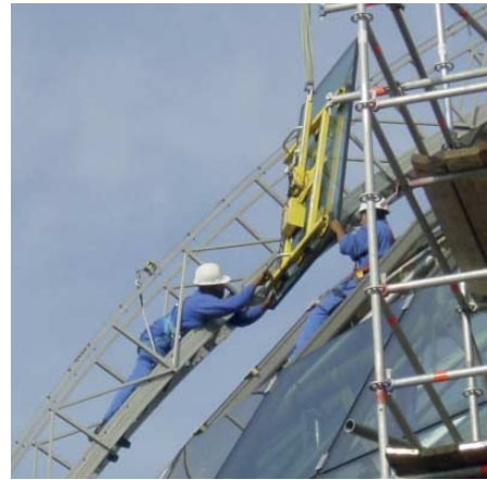
FIG. 176 Installation of the glass panels with usage of the maintenance bridges
