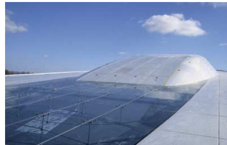
FIG. 187 Completion of the roof
