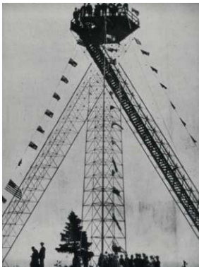
FIG. 19 The outlook tower by Alexander Graham Bell, [1907] as the first 3D industrialized space truss structure
