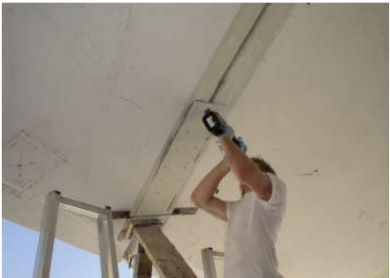
FIG. 155 Assembly of the roof segments by gluing
