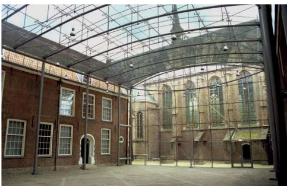
FIG. 84 Glass roof and façade, both with glued connections in the Prinsenhof in Delft in 1996
