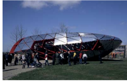
FIG. 224 Exterior of the pavilion (under construction)
