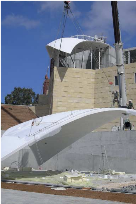
FIG. 154 Preparation and hoisting of the upper and lower wing of the Library in August 2005
