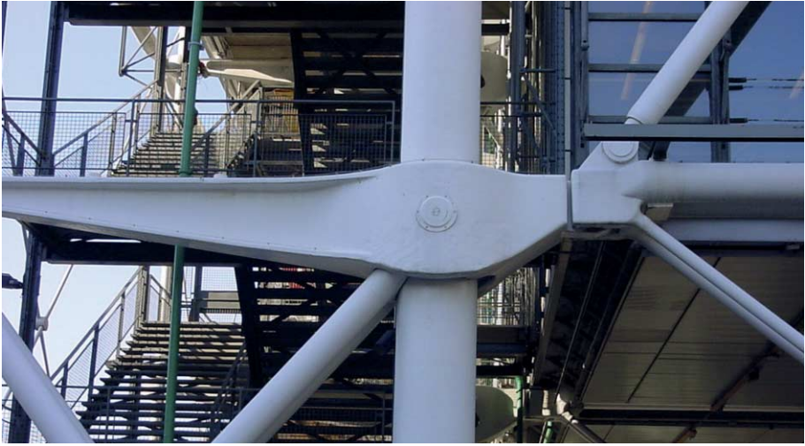
FIG. 16 Detail of the Pompidou Center in Paris.
