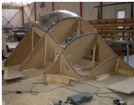
FIG. 130 Fitting of a panel on a mould
