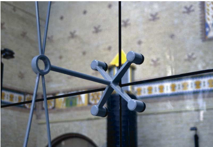
FIG. 64 Detail of the frameless glazing
