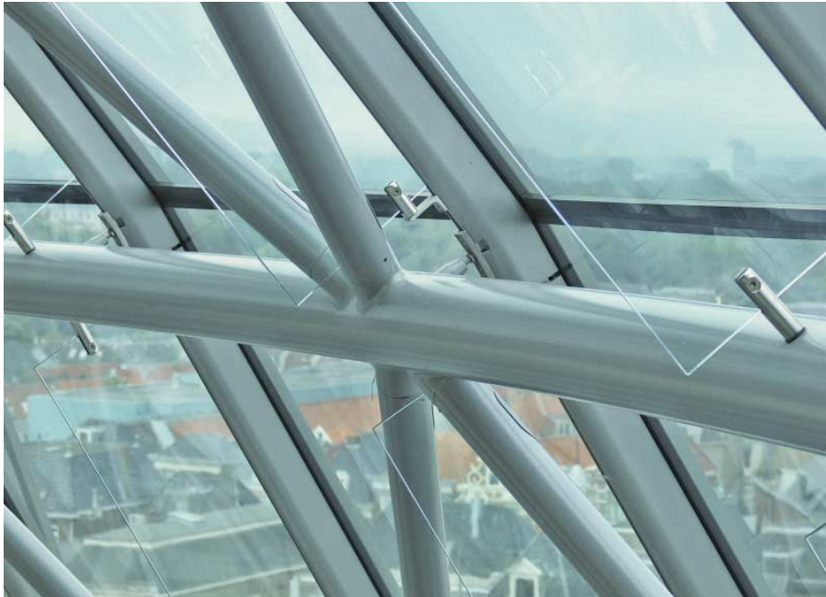
FIG. 174 Connection of an elliptical hollow aluminium glass-profile to the streamlined space frame
