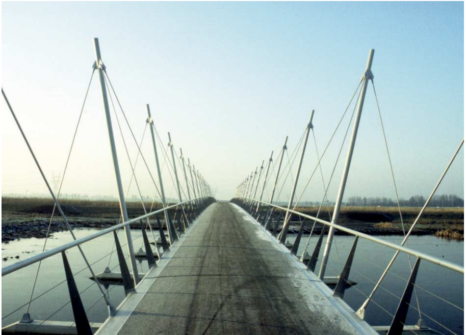
FIG. 197 Tensegrity Bridge in Purmerend
