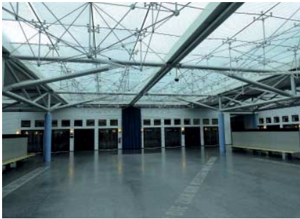
FIG. 82 Lower perspective of first glued insulated glass panel roof in 1995 (Gerard Passchier arch)
