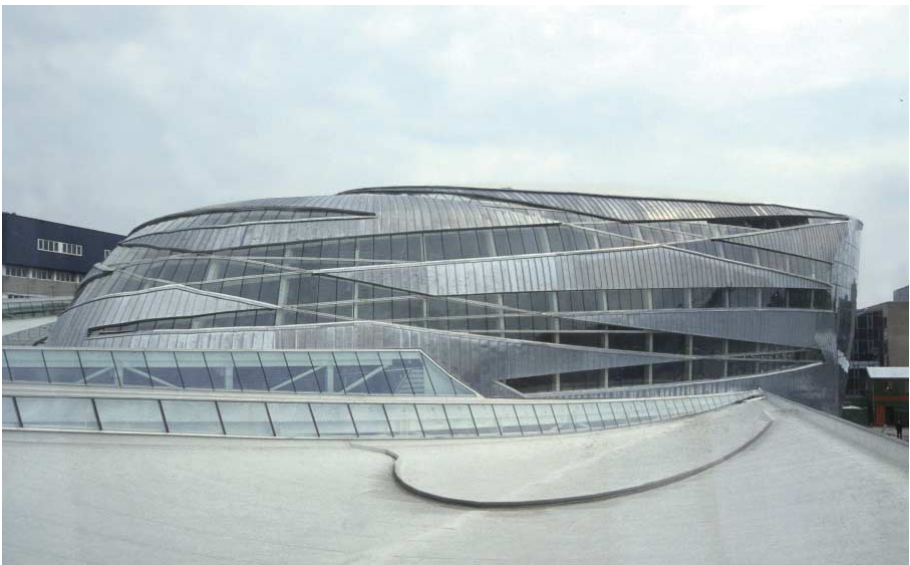
FIG. 108 Construction phase of spaghetti facade with cold twisted glass in the Town Hall of Alphen a/d Rijn.
