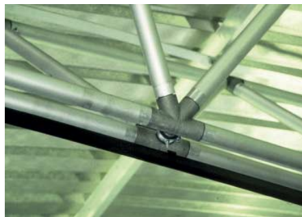
FIG. 208 Node of the space frame
