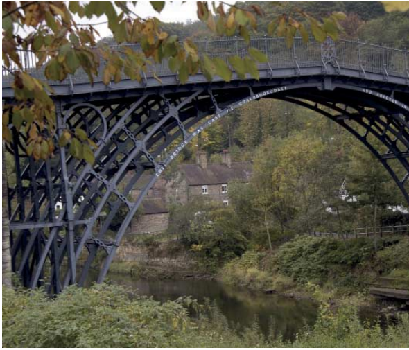
FIG. 17 The iron bridge of Coalbrookdale still stands as one of the early and firm examples of structural cast iron.
