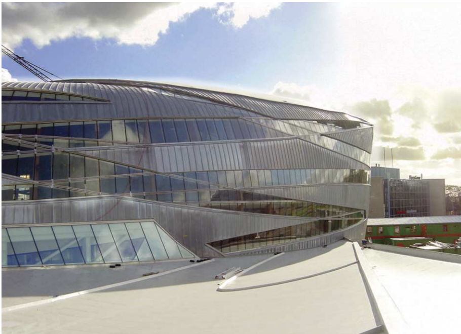
FIG. 239 The 'spaghetti' glass strips with cold twisted glass
