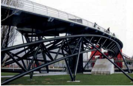
FIG. 34 Pedestrian Bridge in Parc de la Villette in Paris
