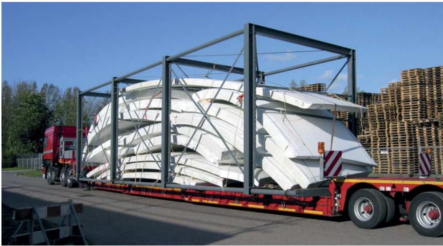
FIG. 153 Open container at Holland Composites with the roof segments ready for shipment in April 2005
