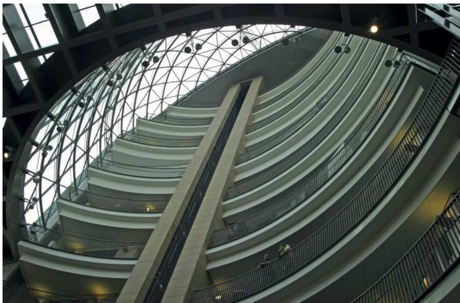
FIG. 177 The roof of the courtyard is suspended from the dome
