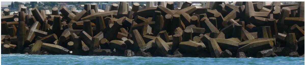
Figure J.4: Dolos Breakwater
