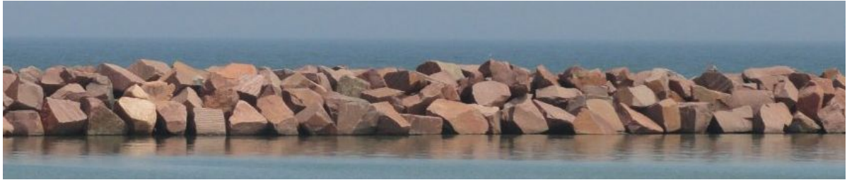
Figure I.1: Rubble Mound Breakwater (JohnsonMatel. (2011). World-Wide-Matel . Retrieved from http://johnsonmatel.com/ . Accessed on November 6, 2014.)
