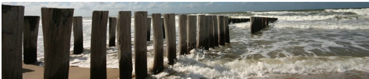
Figure I.17: Timber Pile Breakwater
