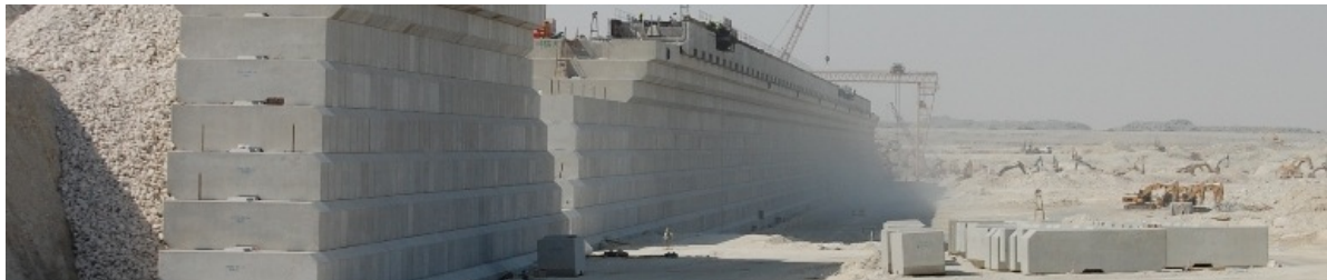
Figure I.11: Block Wall Quay Wall
