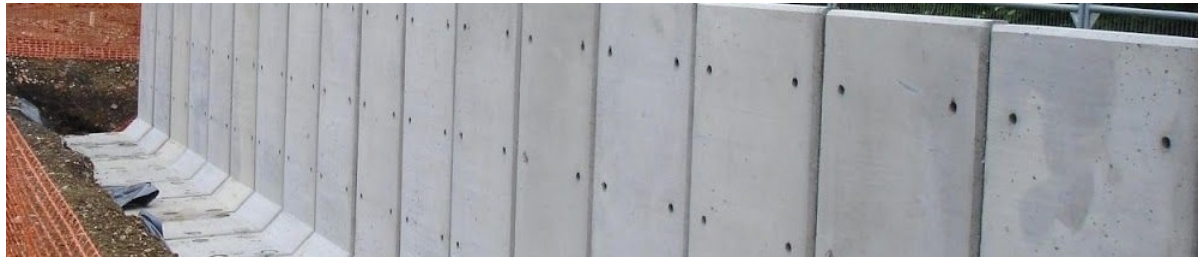
Figure J.5: Concrete L-wall Breakwater
