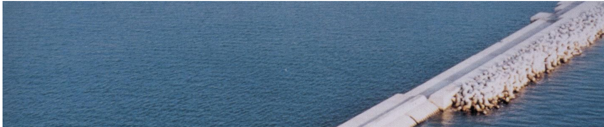
Figure J.9: Horizontally Composite Breakwater (The Liverpool Thessaloniki Network, 1996)
