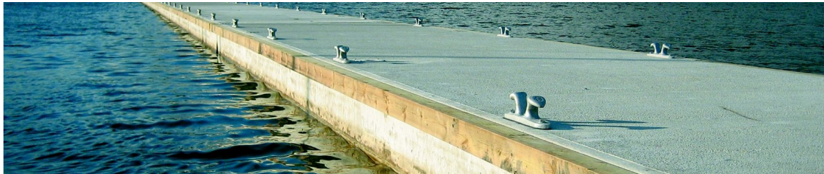
Figure I.14: Floating Breakwater
