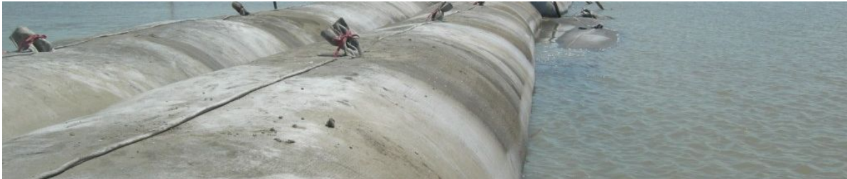
Figure I.33: Geotube Breakwater
