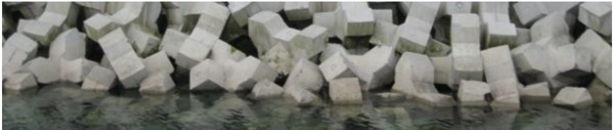
Figure J.3: Xbloc Breakwater
