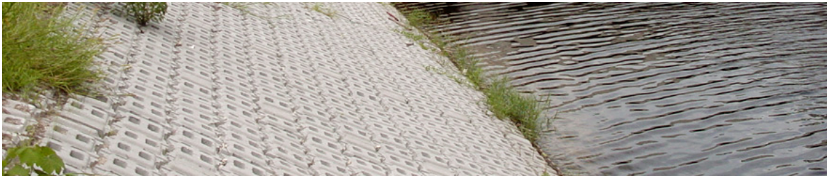
Figure I.3: Armorflex Breakwater
