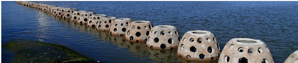
Figure I.24: Reef Ball Breakwater
