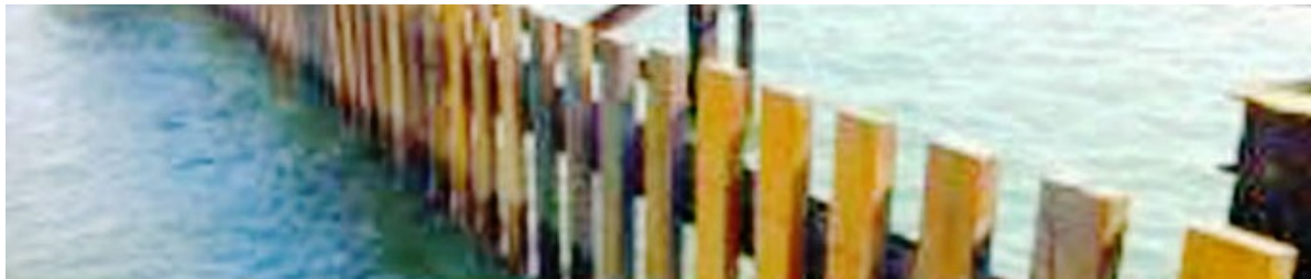
Figure I.29: Screen Breakwater
