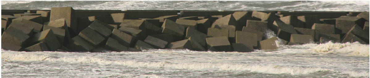
Figure J.1: Cube Breakwater
