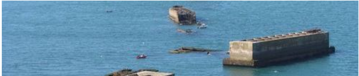
Figure I.8: Caisson Breakwater
