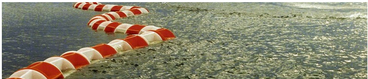
Figure I.38: WaveEater Breakwater
