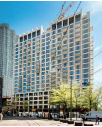
Wijnhavenkwartier, 1975 transformed in 2016, height 73m
