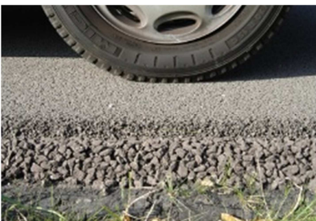
Fig.5.1 Double layered ZOAB or Very Quiet Asphalt(Crow,2012)
