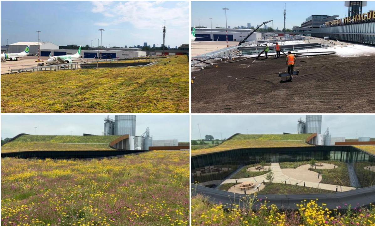
**Figure 2.3:** Real scale green roof system applications by Sempergreen in Europe. *Upper:* Installation of an extensive lightweight traditional sedum system for the terminal of Rotterdam The Hague Airport, the Netherlands - Sustainable expansion project, carried out in 2020. *Lower:* Installation of a biodiverse system on the roof of a factory in Belgium (pictures retrieved online from Sempergreen).
