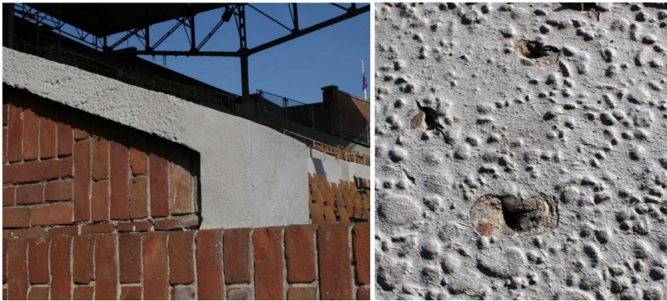
Fig. 1. Example of an aesthetically incompatible repair of historic concrete. Left: Due to a monochrome, grey layer of paint and local smooth repair, the original colour and textural scheme of brickwork and concrete is impeded. Right: Close up of the surface; where the paint has detached, the original polychrome surface influenced by the gravel and cement is visible (Olympic stadium Amsterdam, architect J. Wils, 1928).
