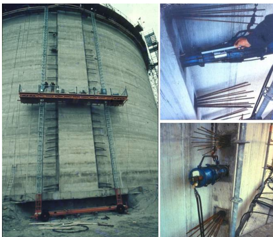
Figure 64 Prestressing LPG Tank Terneuzen (NL) (R. Braam, 2010)
