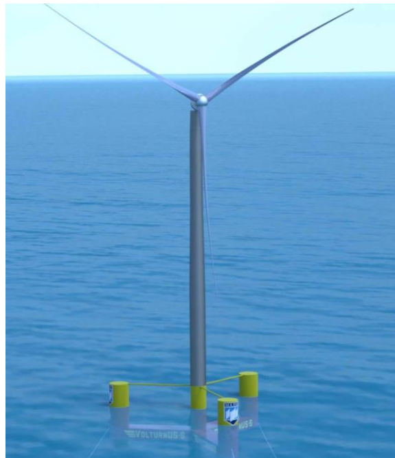
Figure 3.3: The UMaine VoltturnUS-S reference floating offshore wind turbine (Allen et al. 2020).
