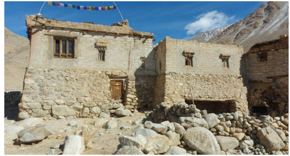
Old abandoned house of Kulum village.
