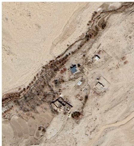
Lower Village | Inhabited and more modern construction because of road access
