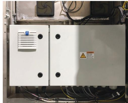
Figure 34. AC charging and Media components enclosure
