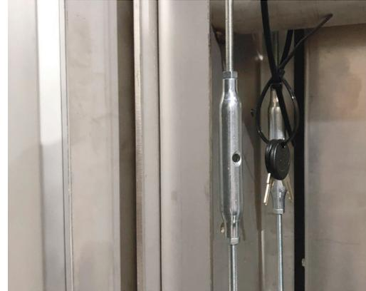
Figure 41. Unnecessary use of stainless steel
