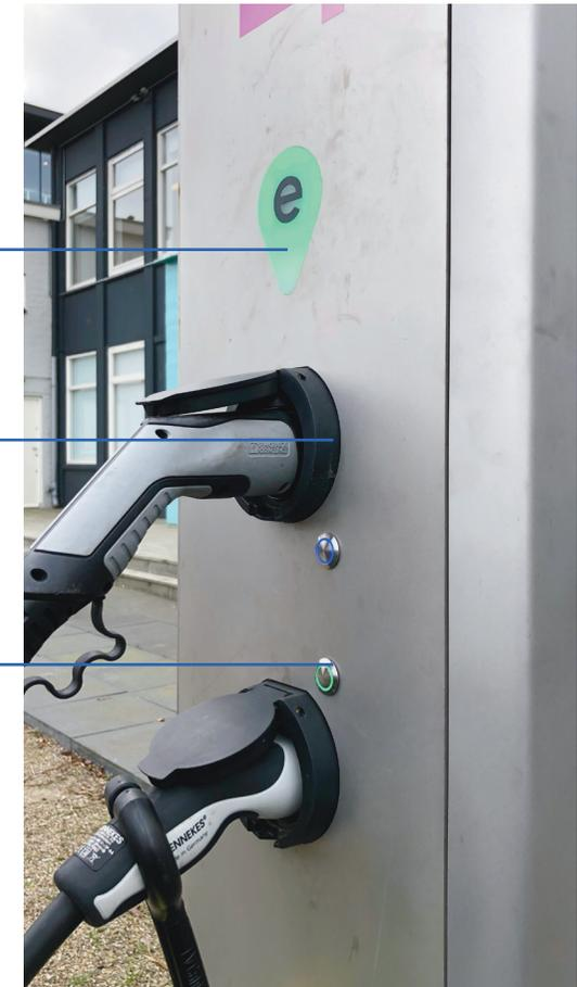
Figure 49. AC charging interface components
