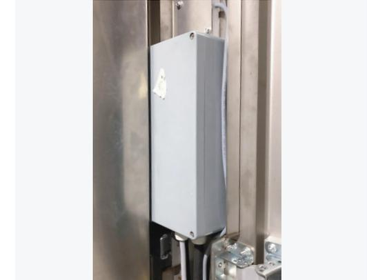
Figure 33. AC sockets enclosure
