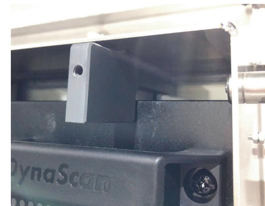
Figure 48. Special clamp to secure the media screen
