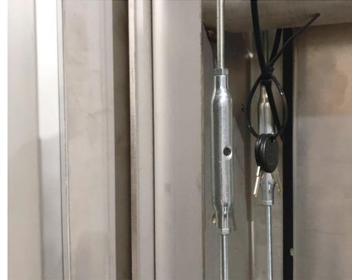
Figure 41. Unnecessary use of stainless steel
