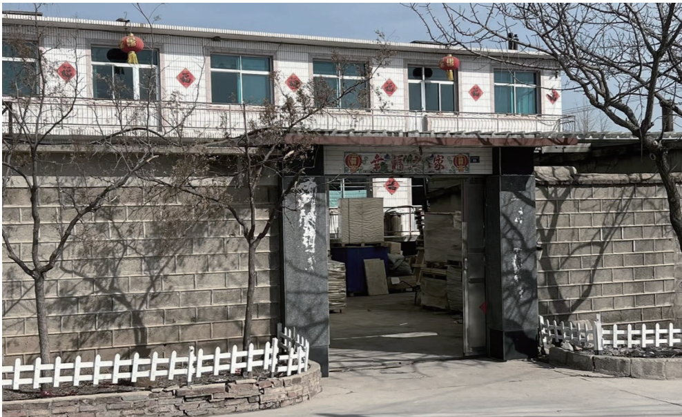
House in good condition Photographed by author
