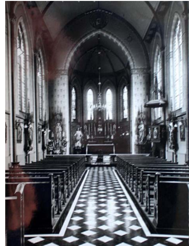
Figure 19. The second interior, date unknown
