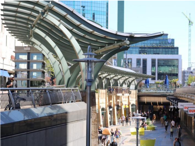
Arched steel canopy spanning the underground passage
