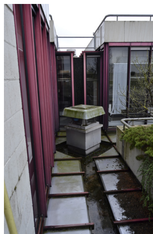
Fig. 2.6.6-2 Here we can see how the rain gutter and ventilator are integrated together. (M.Wang, 2017)
