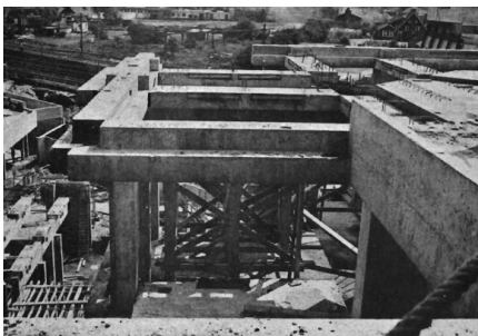
Fig.2.3.31 prefabricated component construction, source from Dokumentatie bouwtechniek 1971
