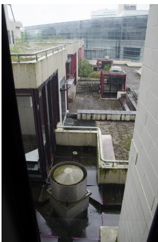
Fig. 2.6.6-1 Ventilator on the roof. We can see there are moss on its surface, which means the outdoor environment is very moist. (M.Wang, 2017)
