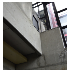
Fig.2.5.20 From some special tower, we can see the clear sign of leaking, also the flat glass roof make water difficult to run away thus cause the problem of moss.(M.Wang,2017 )
