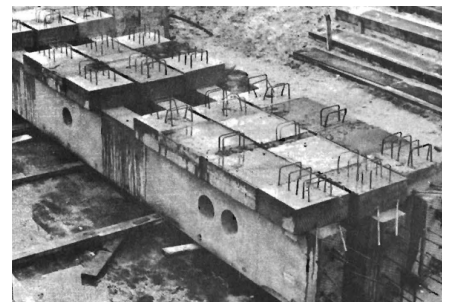
Fig.2.3.31 prefabricated component construction, source from Dokumentatie bouwtechniek 1971
