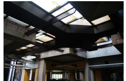
Fig.2.5.14 Look from interior, as the drainage system is designed translucent for where skylight comes in, moss covered some light and the gutter was (M.Wang, 2017)
