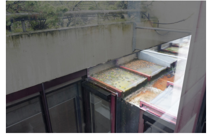
Fig.2.5.12 Moss on the higher drainage gutter surface, and some sign of corrosion on the lower gutter. (M.Wang, 2017)
