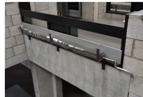
Fig.2.6.9 Heater exposed in the atrium. (M.Wang, 2017)
