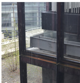
Fig.2.5.19 From the picture we can see the moss on the frame and also on the interior facade which means the facade is not well-sealed to prevent water get in.(M.Wang,2017 )
