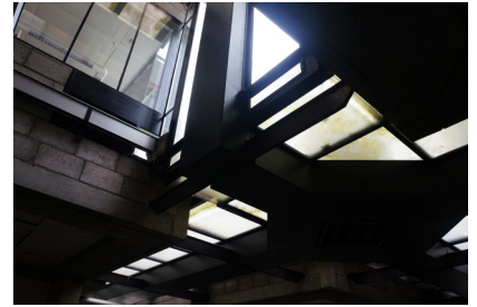
Fig.2.5.13 Look from interior, connection gutter where rain runs from higher "tower" to a lower one. Delicate detail design, but easy to broken with leaking problem. (M.Wang, 2017)
