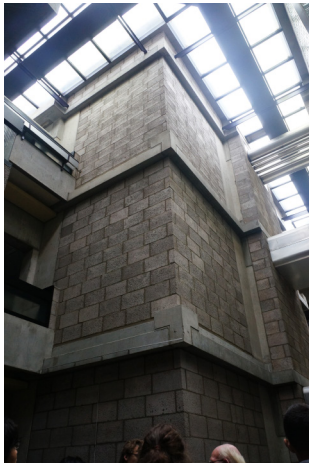
Fig.2.6.8 The concrete block made the building hard to heat during winter and slow to radiate during summer. (M.Wang, 2017)
