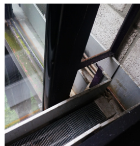
Fig.2.5.19 From the picture we can see the moss on the frame and also on the interior facade which means the facade is not well-sealed to prevent water get in.(M.Wang,2017 )
