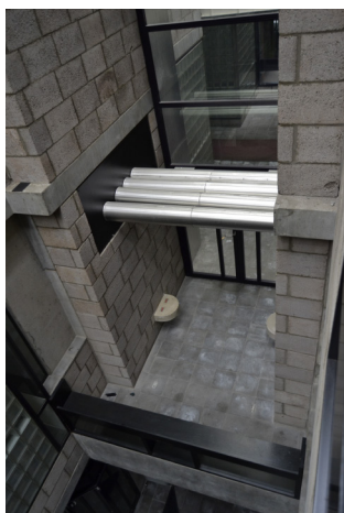
Fig.2.6.10 Left: Heating tubes between different building blocks (picture taken in the interior "street") (M.Wang, 2017) Right: Heating tubes within one building block (M.Wang, 2017)
